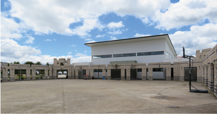
FIGURE 7.9 Courtyard with view to Mosque, Canberra Islamic Centre, Monash, Canberra, 2022
