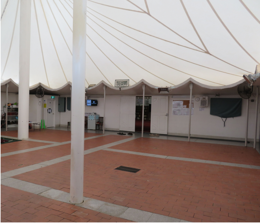
FIGURE 7.18 Interior of the Yarralumla Mosque courtyard, Canberra, in 2022. Interior of the Yarralumla Mosque courtyard, Canberra, in 2022, showing inverted concrete shells which differ from the initial concept by Block, and the more recent sail structures.
