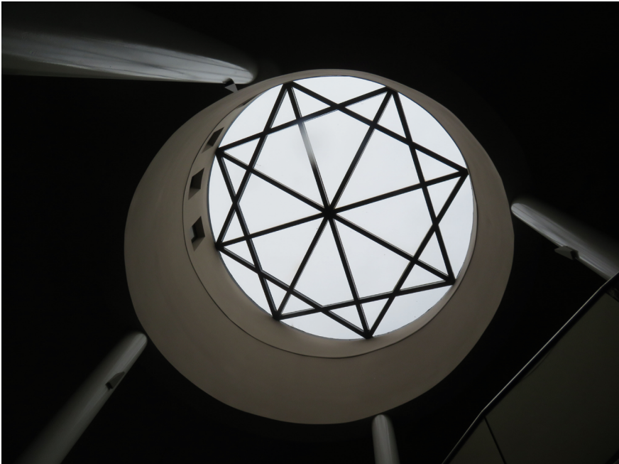
FIGURE 7.14 Skylight at Gungahlin Mosque, Canberra, 2022 PHOTOGRAPH BY MD. M. RASHID
