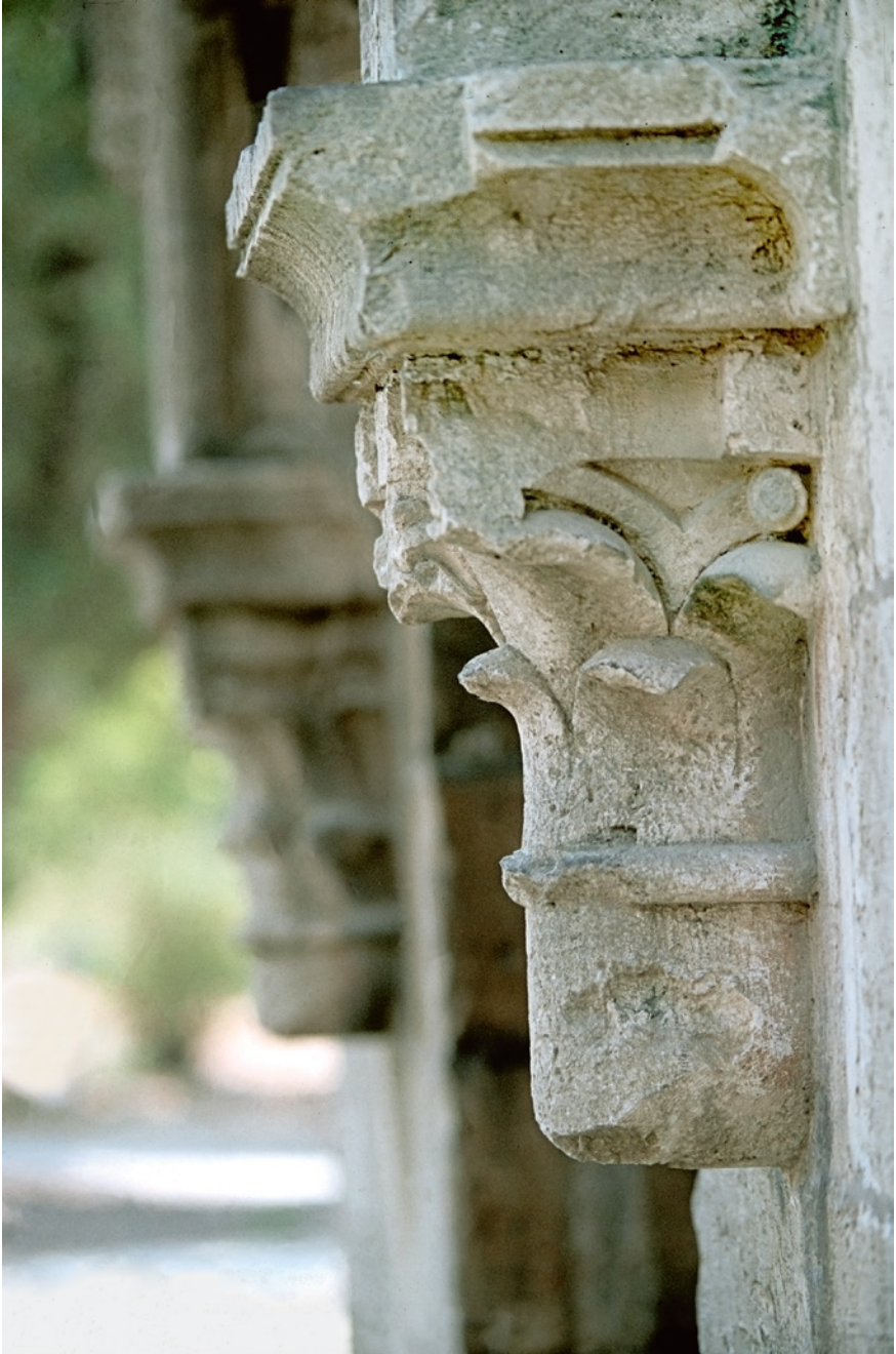
FIGURE 13.4 The Kubakiyya mausoleum (turba), Jerusalem (1289/688): Elbow columns. PICTURE TAKEN BY DEKEL EDUT.
