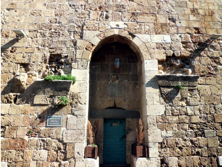
FIGURE 16.2 Entrance to Burj al-Sulṭān. PICTURE TAKEN BY REUVEN AMITAI.
