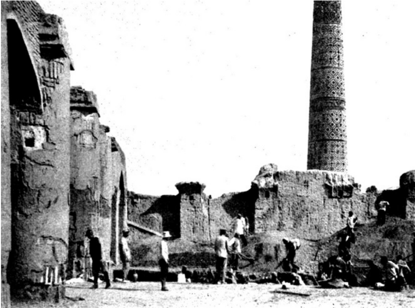
FIGURE 5.2 Schmidt's excavations in the Tari (Tarikh) Khana mosque (AFTER SCHMIDT 1937, FIG. 9).
