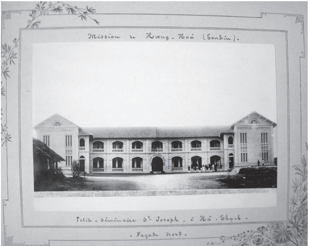
25. North face of the MEP St-Joseph Minor Seminary in Ha-thach, Upper Tonkin vicariate. The seminary was destroyed, along with the buildings of the vicariate's see in Hung Hoa, during the First Indochina War (1945-1954). Undated. Source: MEP Archives.
