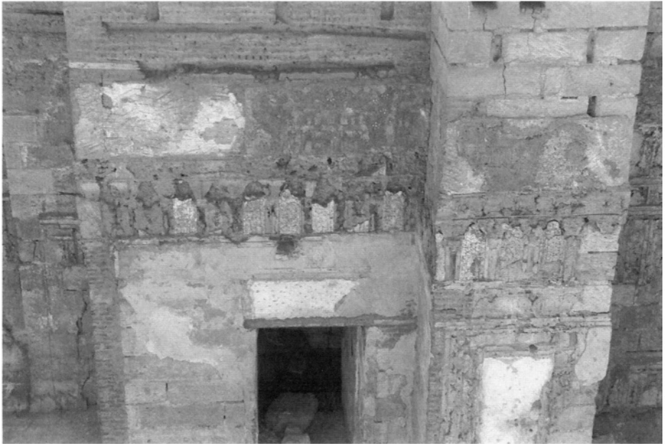
18. The two glass mosaic fragments and the remains of decoration around them in the Qā'a al-Ashrafiyya
