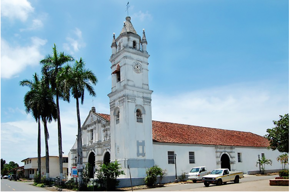
FIGURE 49 Church of San Atanasio, Villa de los Santos, Panama. In this case, we can see how the façade, designed following European architectural trends it's like a curtain that only covers the front of a building entirely designed following the hybrid Native-Ibero-Arab system.
