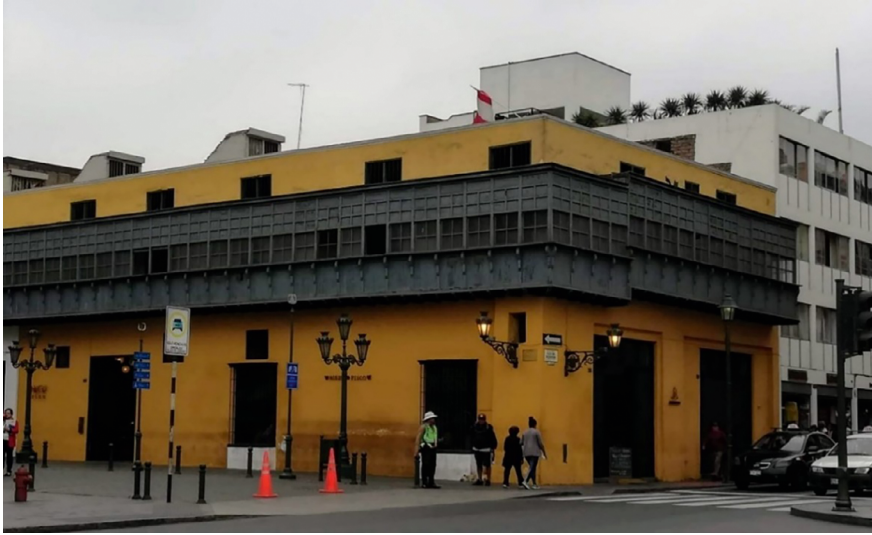
FIGURE 17 Corner balcony, del Oidor House, Lima
