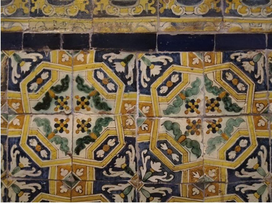
FIGURE 10 Tiles plinths at the Convent of San Francisco, Quito. We can see here a detail of the tile motifs that combine geometric structures and floral designs.
