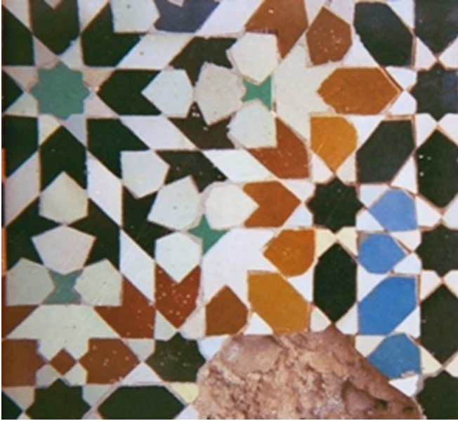
FIGURE 1 A detail of a tile based on the geometric small tesserae in Bin Yūsuf's Madrasa, Marrakech. As the tile is broken, we can see how the complex pattern is composed of a huge number of small pieces.
