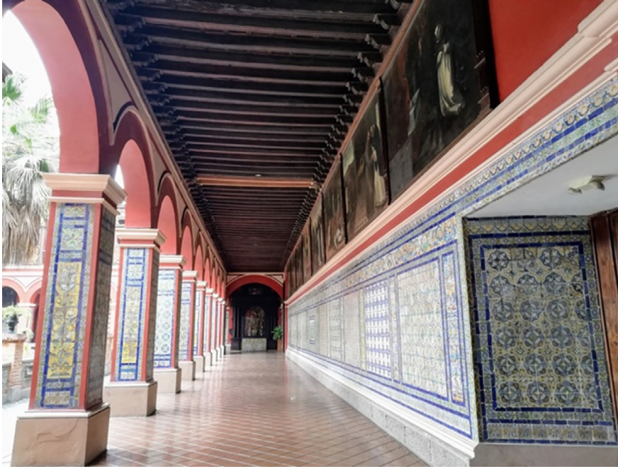
FIGURE 8 Tile plinth at the Convent of Santo Domingo, Lima. We can see here an almost identical tile system (proportions, patterns, motifs, techniques) as we saw in contemporary Tunisia (with the only difference of the Christian or Muslim motives).
