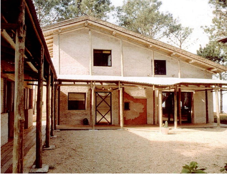
FIGURE 32 El Arca House, Maldonado, Uruguay, by the architect Giancarlo Puppo CREDIT: PHOTOGRAPH TAKEN BY GIANCARLO PUPPO – “GIANCARLO PUPPO – UNA ARQUITECTURA DE LA PLURALIDAD” SOMOSUR XIX – ESCALA, COLOMBIA, MÉXICO, PUERTO RICO AND PANAMÁ – 2003 – JULIO CACCIATORE, HUMBERTO ELIASH Y ADRIANA IRIGOYEN’S INTRODUCTION. PAG.158, CC BY-SA 3.0, HTTPS://COMMONS.WIKIMEDIA.ORG/W/INDEX.PHP?CURID=5908220
