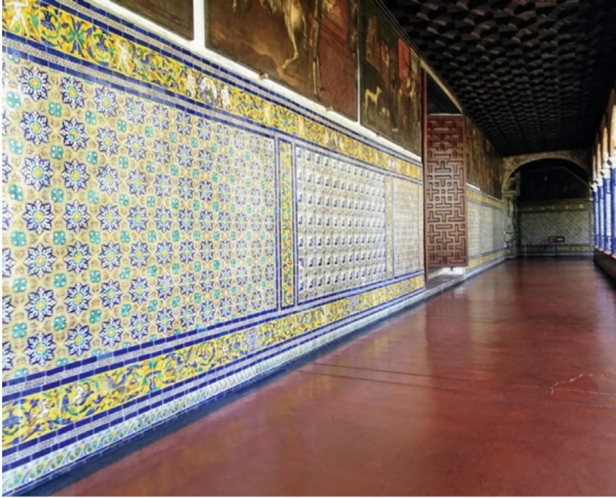
FIGURE 7 Tile plinth at the Convent of San Francisco, Lima
