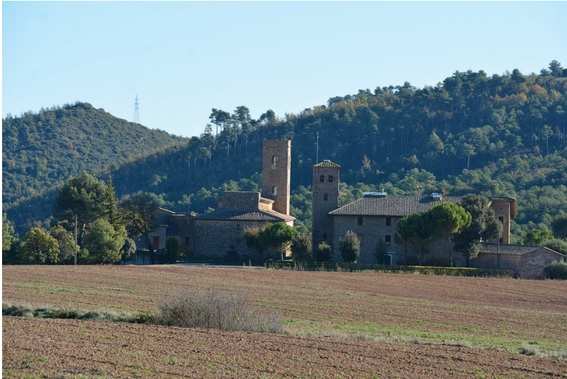
FIGURE 9.2 The nucleus of Bergús from the south, near the disappeared tower of Boixader. On the left is one of the towers under study, Torre Pilota.
