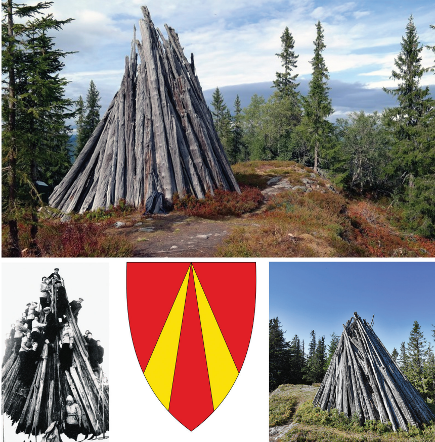
FIGURE 16.1 Vrågåveten in Numedal, c.1807. This beacon is a remnant from the Napoleonic wars. It has become an important symbol, and appears in the municipality's coat of arms. It is 6m high, and 6.5m wide.
