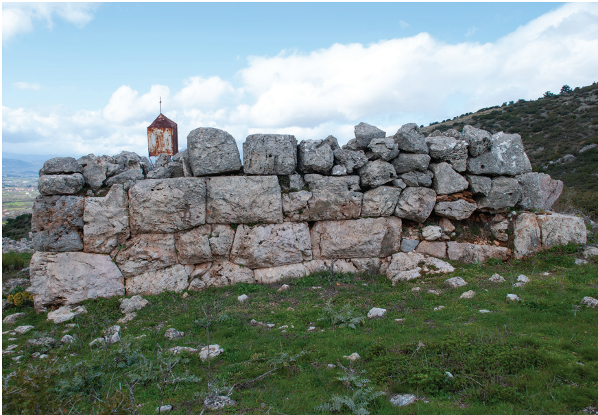
FIGURE 4.6 South-eastern side of the watchtower at Agios Athanasios, where original blocks have been replaced with smaller blocks and tile fragments. A possible doorway can be seen in the eastern corner.
