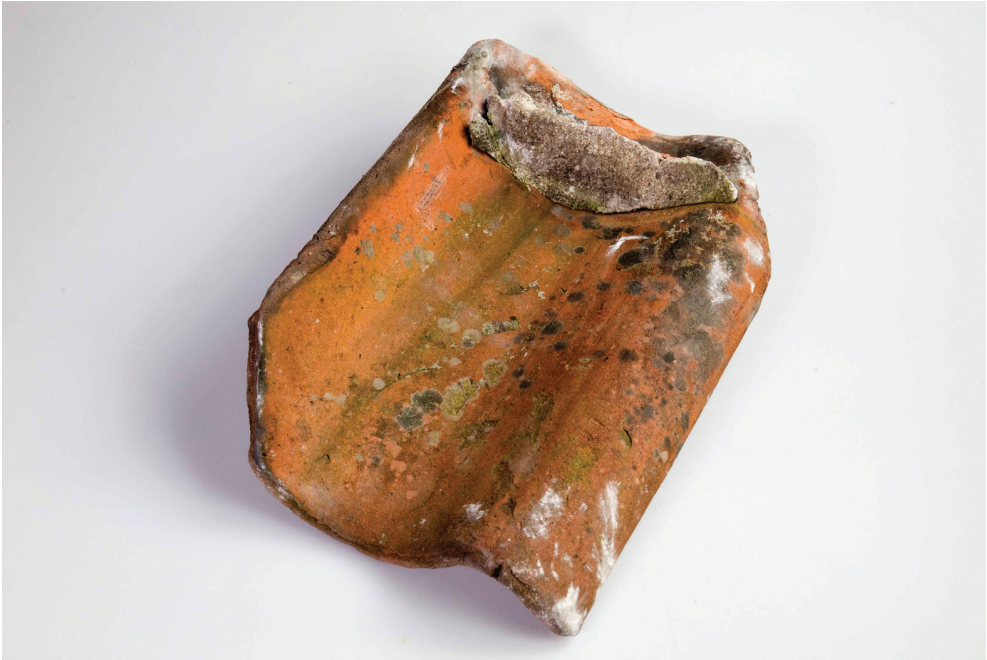
FIGURE 3.1 A red, ceramic tile from the roof of Aalmarkt 11, probably from the sixteenth or seventeenth century. In the fifteenth century, the building had a wooden roof construction covered with slates, but these were replaced with cheaper tiles
