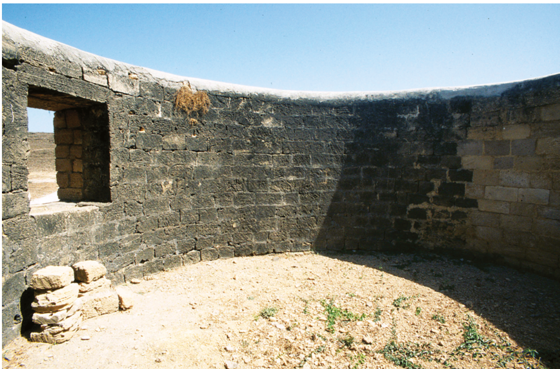
PLATE 5.13 North Tower, interior looking south-east and showing the squat, almost square opening of the entrance, well above the present floor level. Restored stonework can be seen on the right, as well as in the jamb of the entrance.
