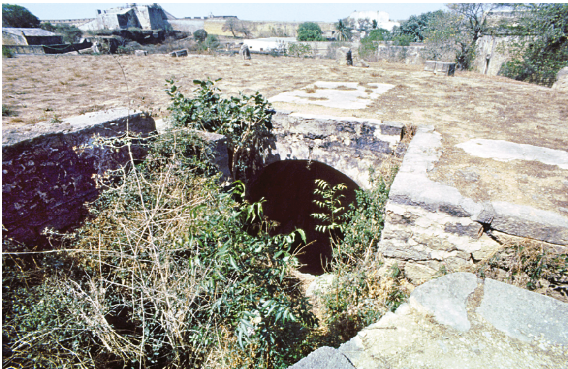
PLATE 3.28 The Queen's Cistern (26) built entirely underground with two or more chambers, view into one of the vaulted chambers.
