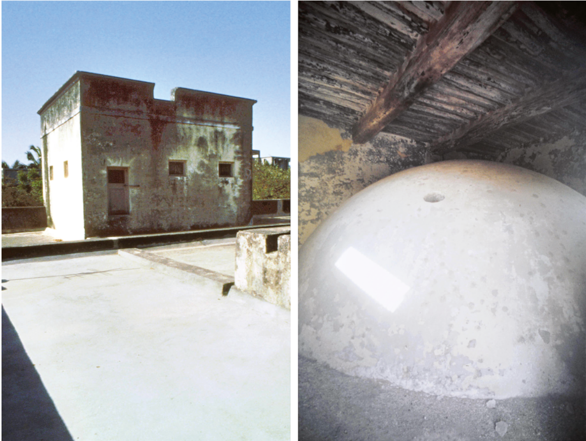
PLATE 5.8 Fire temple. Left: the chamber on the roof concealing the southern dome, exterior view looking south-west and showing the platform of the chamber and the door which provides access for the maintenance of the dome. The gap in the cornice is for ladder access to the roof. Right: the dome of the southern domed chamber (i) as it appears from inside the chamber on the roof which conceals it. The flat ceiling of the chamber can be seen as well as one of the ventilation holes in the dome.
