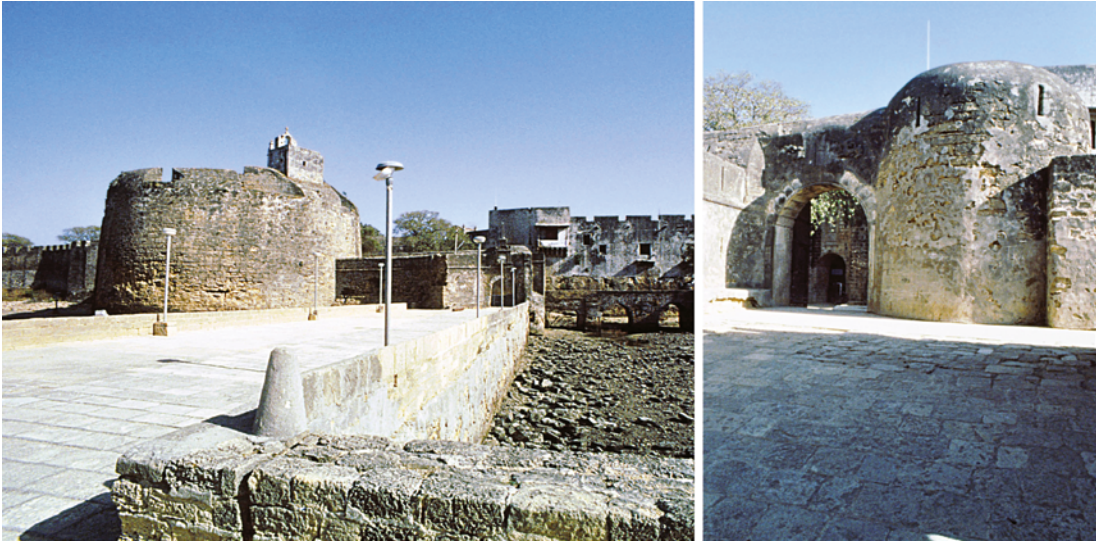
PLATE 3.13 Left: view from the jetty looking south towards the opening of the entrance's outer enclosure, with St George's Tower (19) topped with St George's Chapel to the left and the moat (now dry) to the right, as well as the bridge with three arches. The left arch, which was in a state of disrepair and has since been restored, was originally a drawbridge and the additional arch was not keyed properly into the left pier. Beyond the bridge the outer façade of the Old Governors' Residence (6) can be seen. Right: gate (3) to the forecourt of the main gate, view looking south with an unnumbered tower and the way to the drawbridge on the right. The main gate (5) can be seen in the background through the archway.
