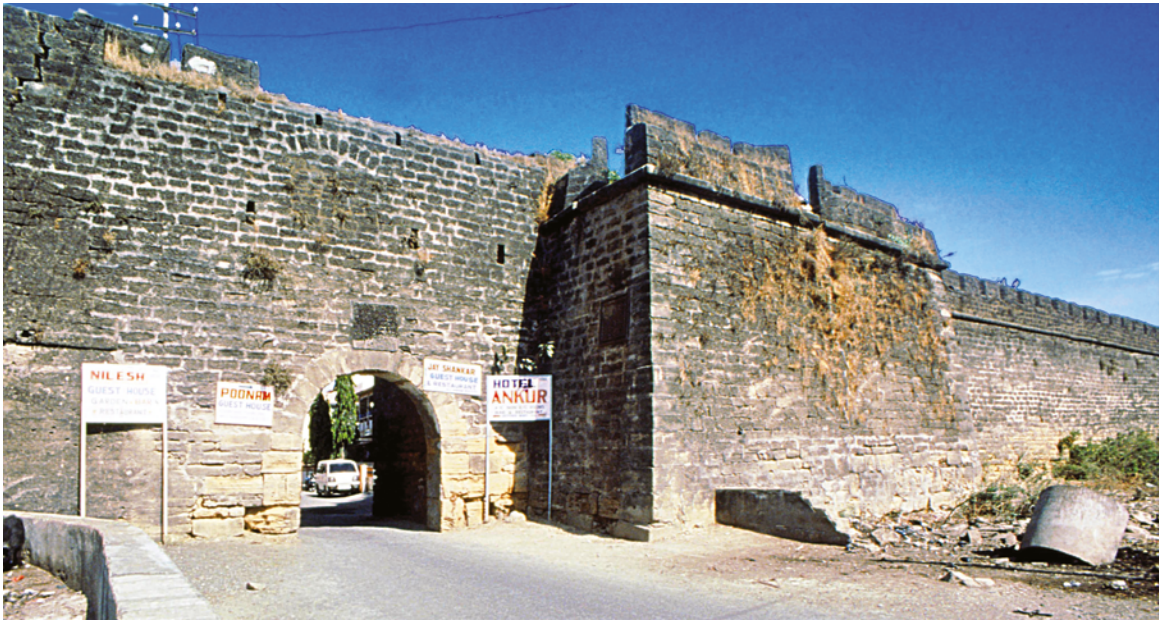
PLATE 4.25 Western town wall, St Peter's Tower (no. 54) and the postern gate to its north seen from outside the town. Above the gate is an arch which has been blocked. The inscribed slab of 1570 over the gate and of 1584 on the north face of the tower can also be seen.
