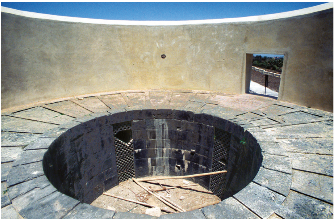
PLATE 5.15 South Tower, interior from the south-west showing the entrance, the pāvis (open coffins for adults and children), the central shaft and two of the drainage ducts faced with pierced stone panels ( jālī ). The aperture giving a view to the sagrī is in the wall to the left of the entrance.
