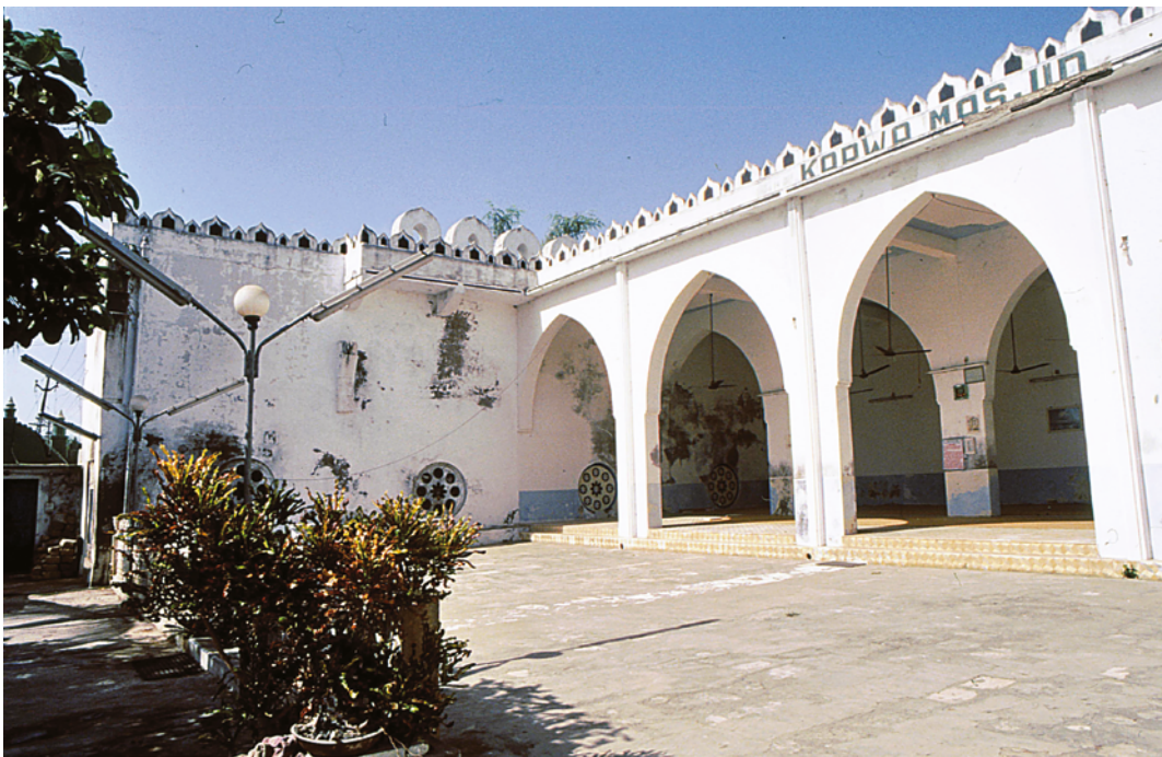
PLATE 4.23 Caravan Masjid, south wall and part of the prayer hall. The high side wall, with its round jālis and the remains of the impost of an arch, enables us to visualise the original form of the prayer hall with its front arcades. Around the roof, the small crenellations seem to have been added to give a finished appearance to the standing prayer hall. However, above the southern wall of the prayer hall some of the old crenellations have survived, conforming in shape and scale to those shown in De Castro's 'map'.
