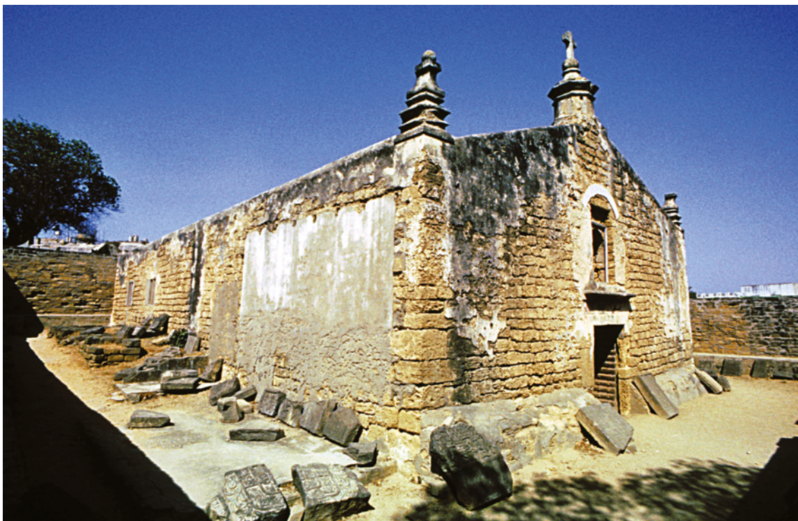
PLATE 3.32 The Powder Magazine (24), exterior view from south-east of the enclosure showing the south and east façades, as well as some of the fragmentary carved or inscribed panels kept in the enclosure.
