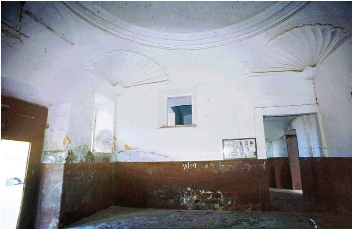
PLATE 4.62 St Paul's Seminary, upper domed room at the eastern side, with the dome standing on squinches constructed in the manner of late and post-Mughal buildings and finished with plasterwork with shell patterns.
