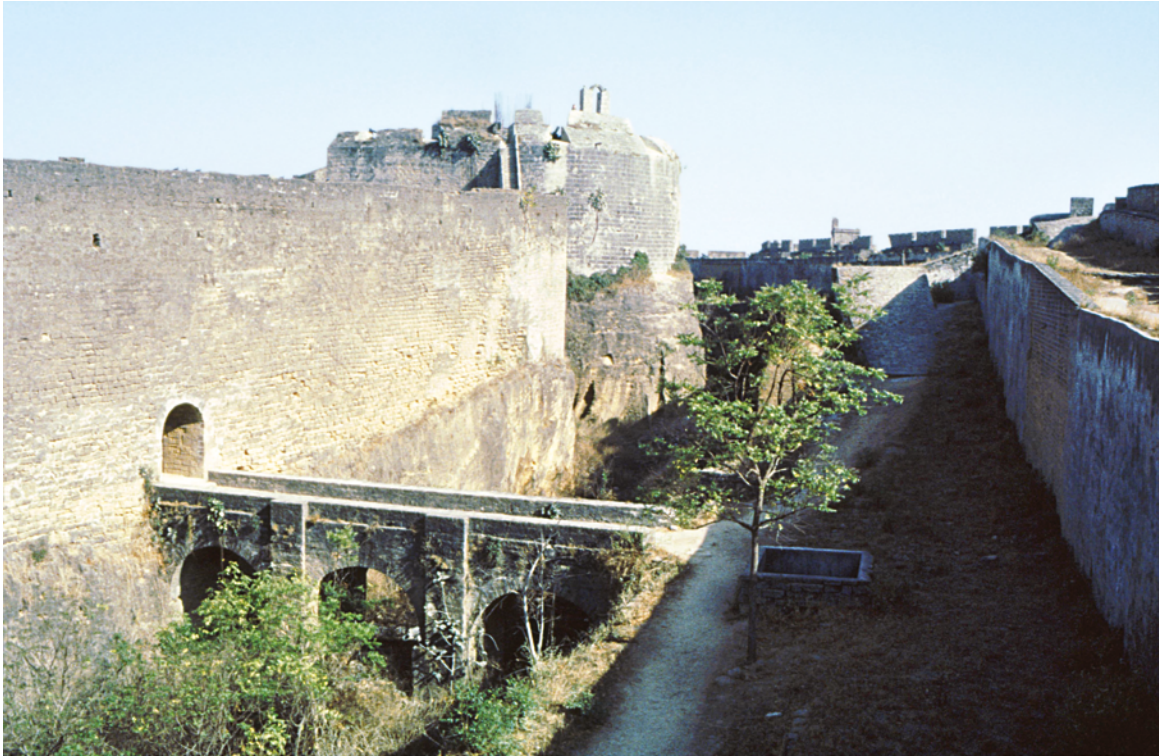
PLATE 3.9 Diu Fort, view from St Dominic's Tower (8) looking south, with the inner walls of 1541–2 to the left and the outer wall of 1546 to the right. Between the walls is a ditch, over which stands the bridge (f) which leads to the postern gate opened after the construction of the outer walls. The gate gives access to the area between the two walls and there is no access to the outside from this area. In the background is the Knight's Tower (11). The location of the older postern gate is behind the Knight's Tower and cannot be seen.
