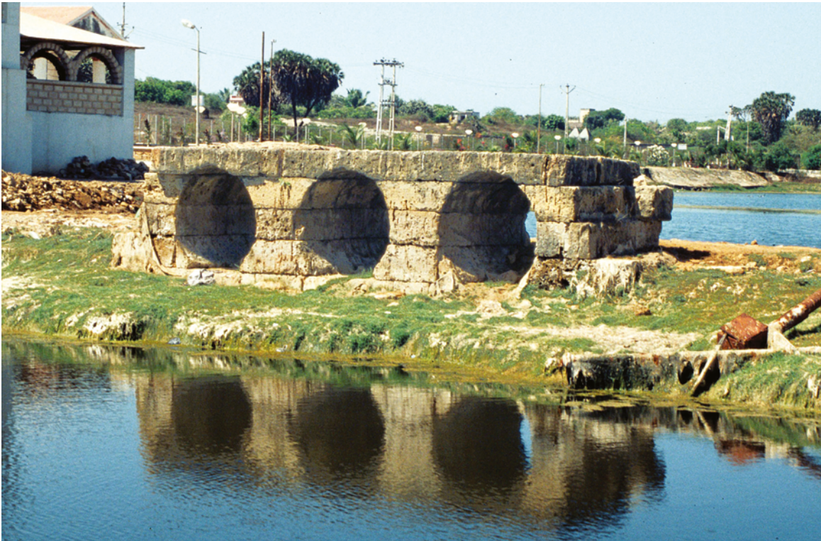
PLATE 6.21 Diu, Dhobi Talao , sluices, view from the reservoir.
