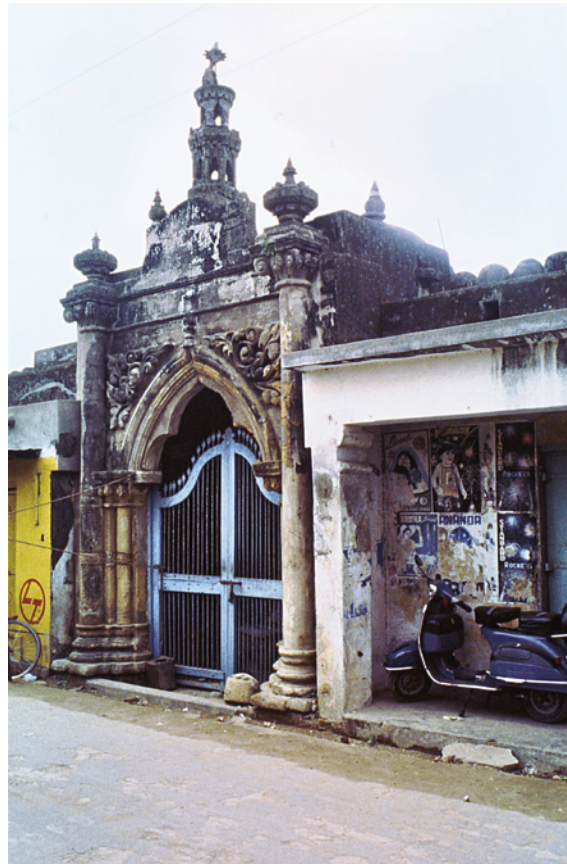
PLATE 4.16 Karao Jāmi', the north entrance, exterior from the south-west showing the Portuguese style of the gate, with pseudo-Ionic columns, a three-lobed arch, finials at the roof level over the arch and topping the columns. The ornamentation, however, depicts nothing which would be objectionable to the Muslims.
