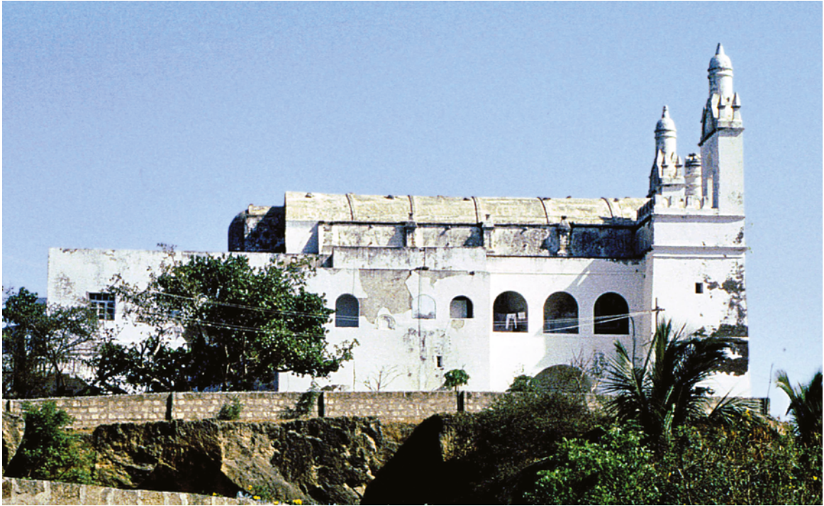
PLATE 4.42 St Thomas's church (81), now Sé Museum, general view from south-east also showing the retaining walls of the southern churchyard.
