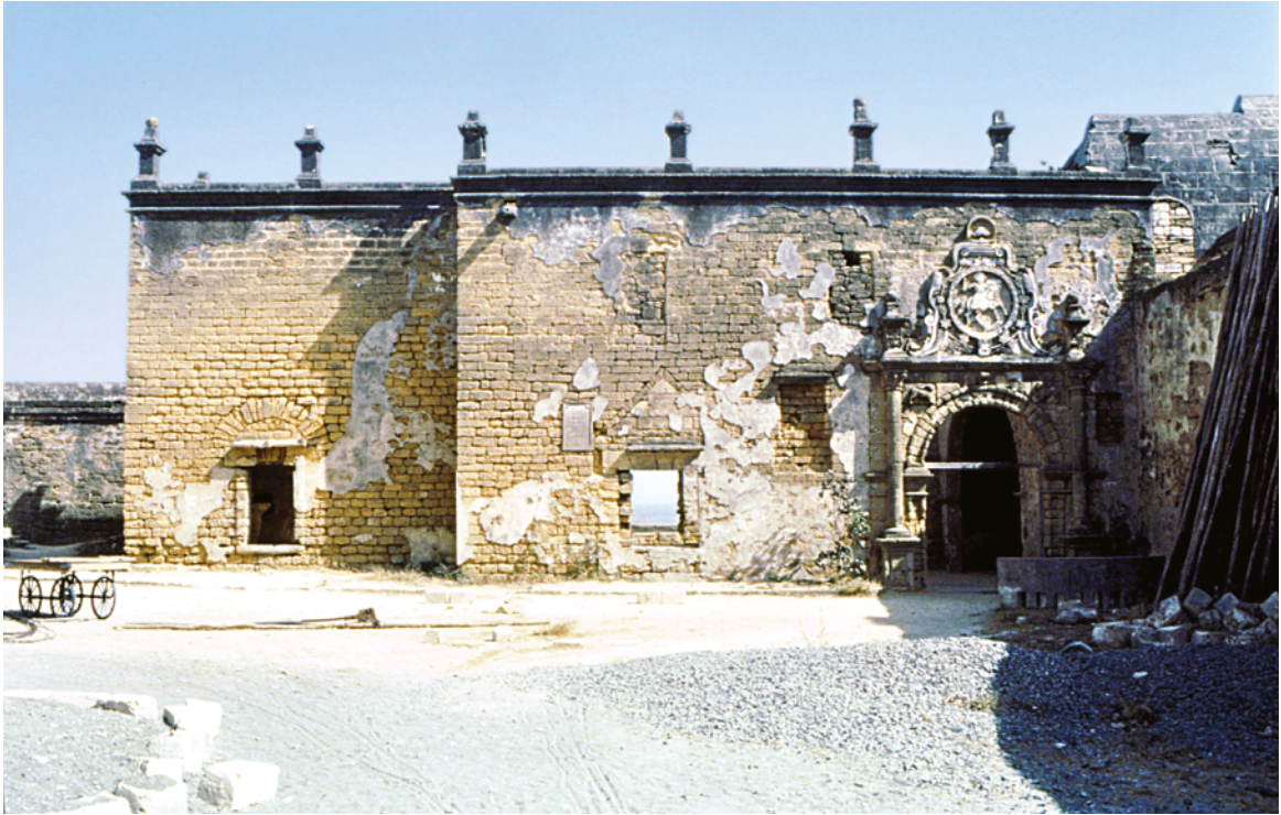
PLATE 3.36 St James's chapel ( Capella de São Thiago , 22), northern elevation also showing the entrance. Some of the plasterwork of the wall has survived including the crest above the entrance. A number of the older windows (now blocked) can also be seen, along with alterations such as a blocked up triangular feature over the open window. To its left is the inscription of 1810.
