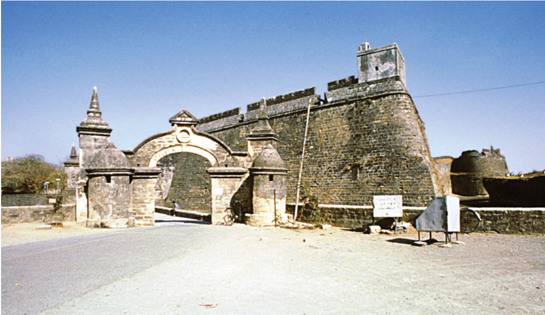
PLATE 3.2 First entrance gate (1) to the fort with the outer wall of 1546 behind. The bulwark in the foreground is St Dominic's (8) and that to the right in the background is St Nicholas's Tower (10). Part of the moat can also be seen. The present arched gate has been reconstructed in later dates.
