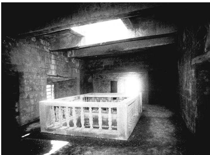
PLATE 3.51 Forte do Mar, chamber below the roof of the keep. The balustrades around the opening in the floor are modern, but the opening, and that in the ceiling to the roof is part of the original design.
