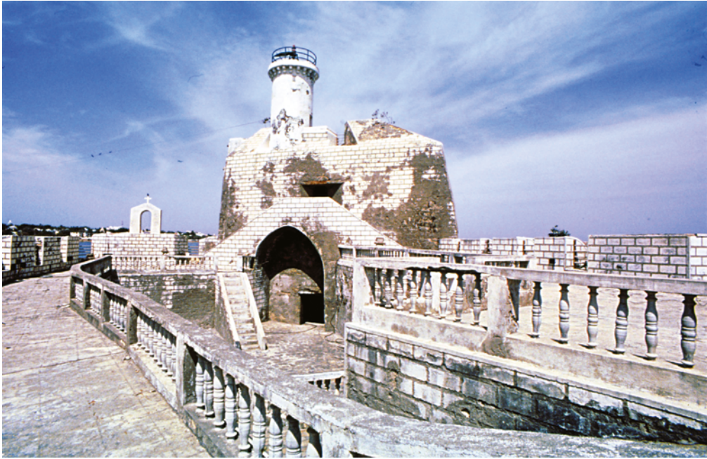
PLATE 3.48 Forte do Mar, south-east court looking north-west towards the keep. The wide arch, along with the steps from the walks, ascending to the opening of the chamber below the keep, are later additions and the opening seems to have originally been an aperture for a cannon. The small opening under the arch is an entrance to the corridor which leads to the north-west yard. The lighthouse on the roof of the keep is fairly modern.
