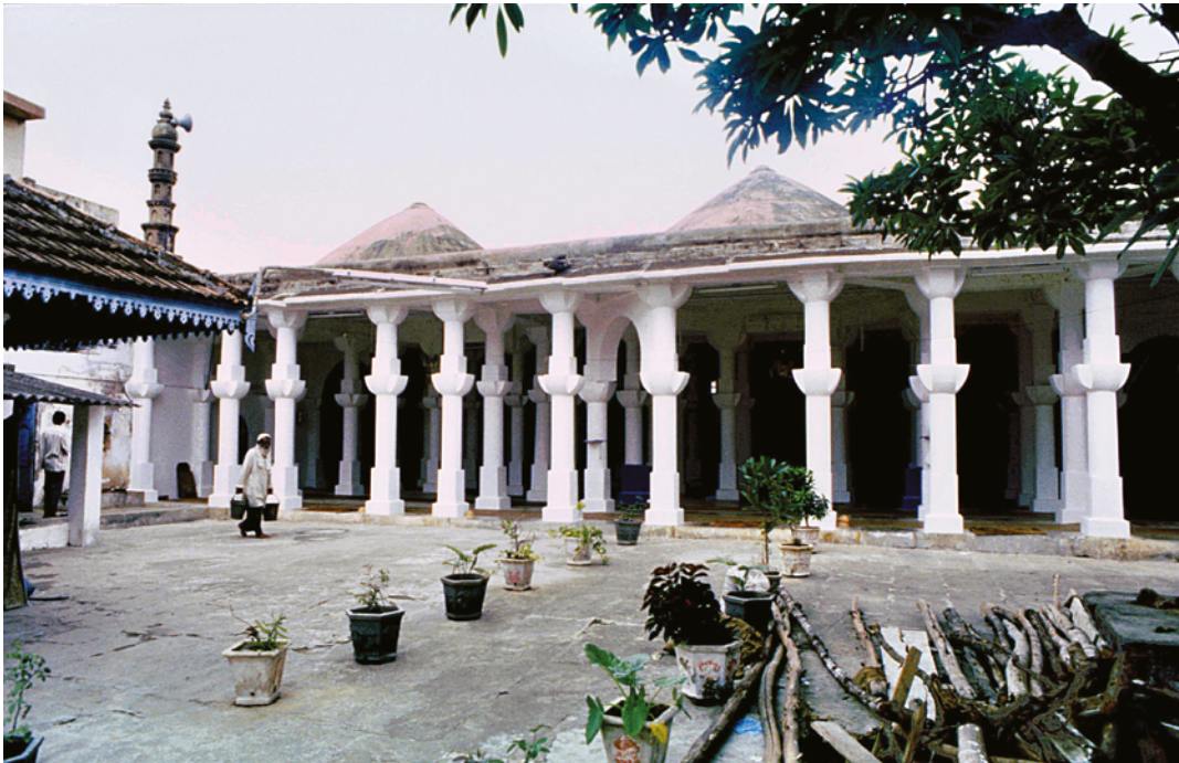
PLATE 4.9 Karao Jāmi', prayer hall, exterior from the courtyard looking east. The columns are each composed of a full-height ancient column together with its bracket capital, superimposed with a short column. These columns do not seem to have been cut to size but are in their original form and height, although their details are now obscured by modern cement plaster.
