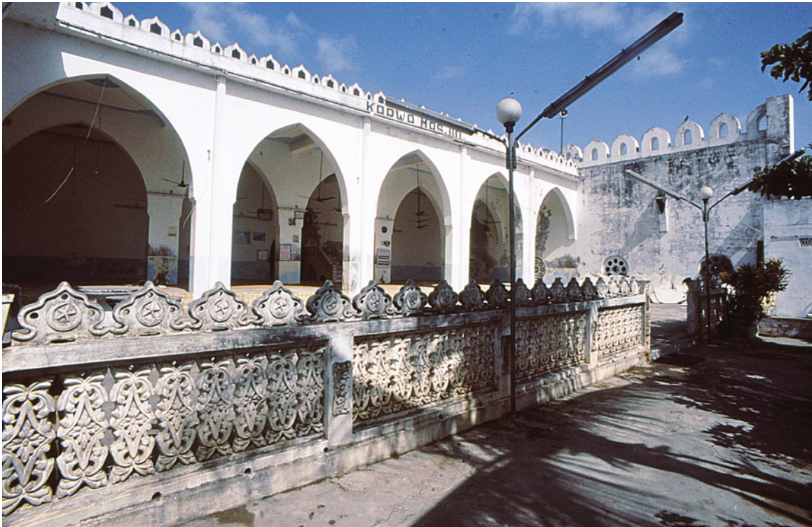
PLATE 4.21 Caravan Masjid (no. 49), prayer hall seen from the south east looking at the five standing bays and the two aisles. The high wall outside the bays is original and was once part of the prayer hall, the impost of a fallen arch and the round pierced stone windows are preserved.
