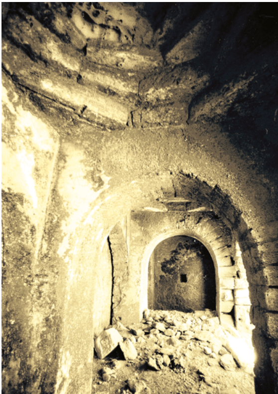
PLATE 6.28 Fudam, old building in the cremation grounds, the standing domed units at the west side of the structure looking north.
