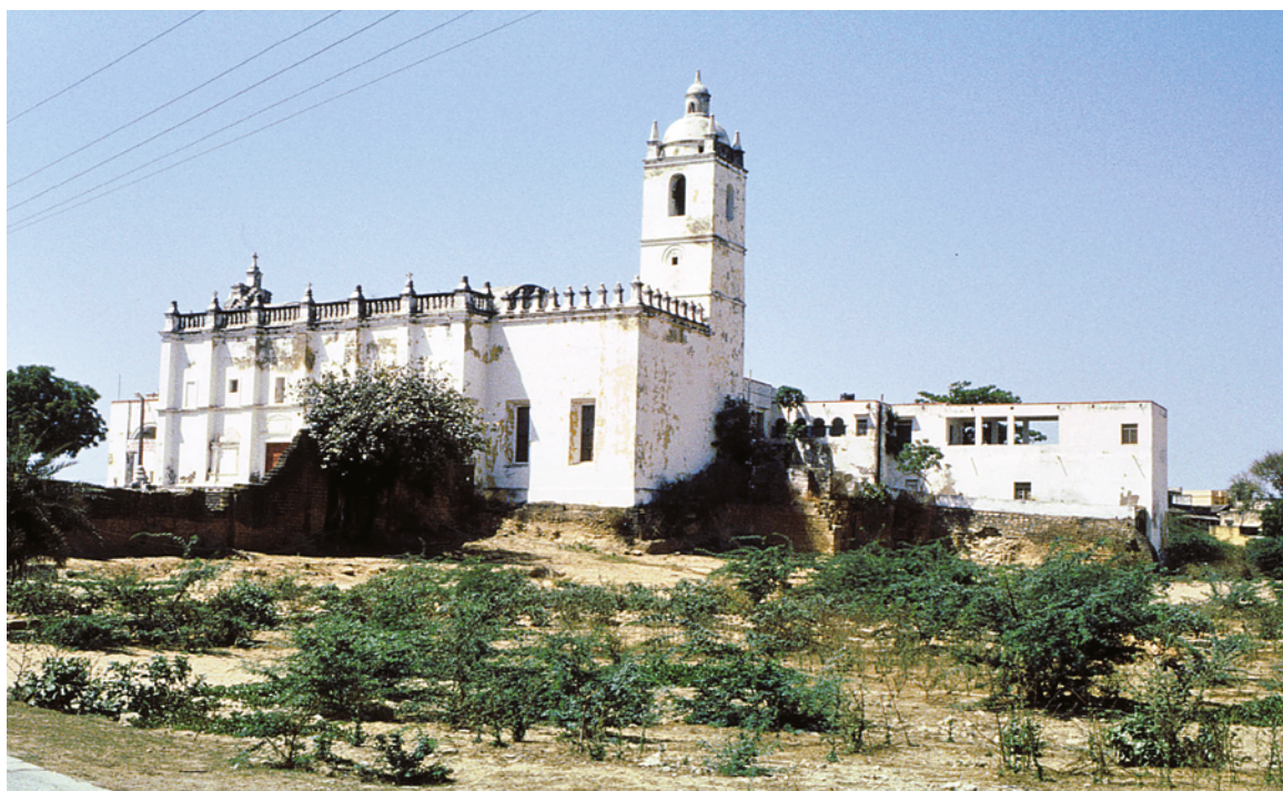
PLATE 4.50 Church and Monastery of St Francis from the north-east. To the left of the belfry of the church the top of the vault of the nave can be seen behind the parapet, but the vault of the choir is not visible. To the right of the belfry is the arched balcony of the monastery. The structures to the far right are modern extensions to the hospital.
