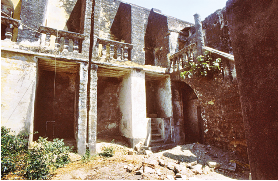
PLATE 6.40 Vanakbara, Church of Our Lady of Mercy, the steps between two of the buttresses on the south exterior of the building, giving access to the pulpit, and above the steps, part of the open walkway passing through the arched openings in the buttresses.
