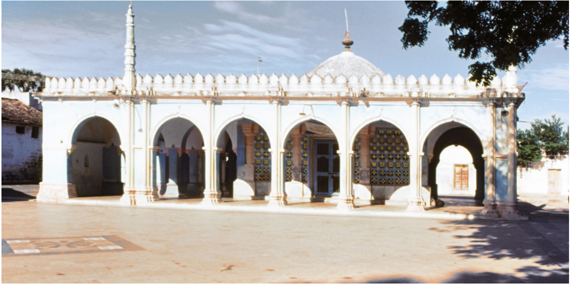
PLATE 2.4 Una, the shrine of Maulāna Shāh Shams al-dīn where Malik Ayāz is recorded to have been buried. The shrine is on the road to Dilwāra and only a few miles from Diu island. The structure with a domed square chamber surrounded by an arcade is traditional for Gujarat, but the extra bay at the left side of the photograph is a later addition. The turrets at the corners of the building signify the extent of the original building.
