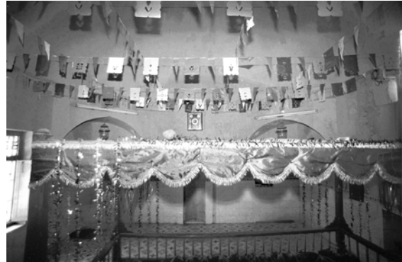
PLATE 6.30 The shrine of Pir Ḥabash Bābā, interior looking west and showing the mihṛāb and two of the squinches built at an unusually low level into the corner of the walls rather than being set over the walls in the conventional way.
