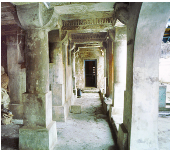
PLATE 4.10 Karao, Jāmi', colonnade to the east of the courtyard. The re-used temple columns are of a standard size and while now plastered over, it seems that they were composed of monolithic shafts in at least two registers, square in plan below and cylindrical above. The upper register could have been fluted or had ornamentation, which has been chopped off. The lintels of the ceiling, which are not plastered over, display their original carving.
