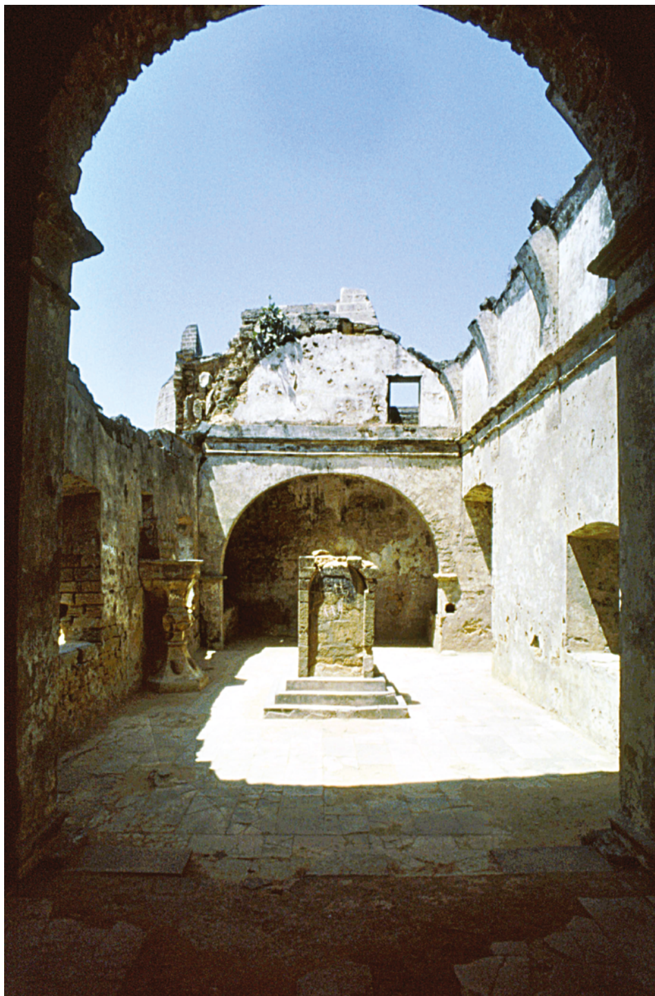
PLATE 3.38 St James's chapel, interior view of the nave from the choir looking west towards the entrance, seen on the right. On the left is the pulpit and high up on the right above the wall part of the vault and two of its re-enforcing arched ribs can be seen. The commemorative pedestal erected in 1906 in the centre of the nave is inscribed with a transcription of an older but undated text found in the ruins of the old cathedral of the fort.
