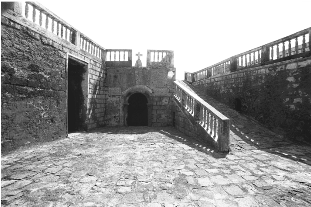
PLATE 3.49 Forte do Mar, south-east court, looking south-east towards the Chapel of Our Lady of Victories and the ramp to the banquette at its right. The opening at the left of the chapel is to a small room, where the Holy Sacrament might have been kept. Both the chapel and the chamber next to it are light in structure and added later.
