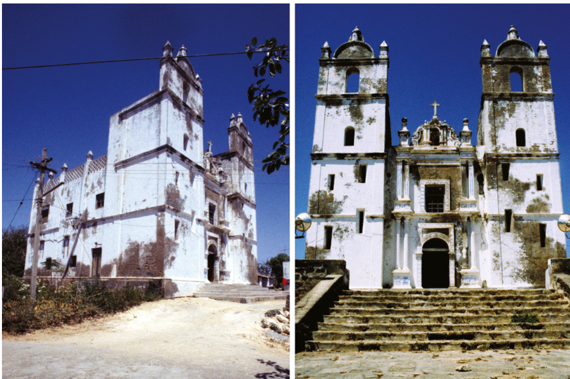
PLATE 6.22 Fudam, Church of Our Lady of Remedies (12). Left: general view from south-east also showing part of the churchyard and the modern ramp to the church terrace. Right: eastern façade with the original steps to the terrace in the foreground.
