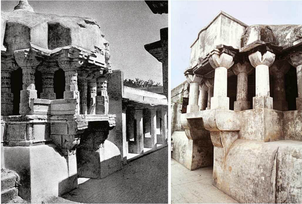
PLATE 4.17 Karao Jāmi', eastern (main) entrance, built of temple spoil with fine carving. It lacks the symmetry of ancient temple entrances, but follows their general plan and structural form. Left: an old photograph. From Marjay, Plate 68. Right: present condition with the carvings plastered over.
