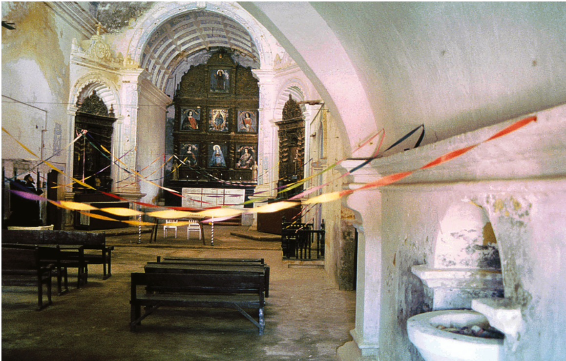
PLATE 4.52 St Francis's Church, interior from the south-east under the vault of the mezzanine, looking north towards the choir and the main altar. The carved altarpieces at either side of the choir can also be seen, set into niches which appear to be later additions and end at the level of the imposts of the choir vault.
