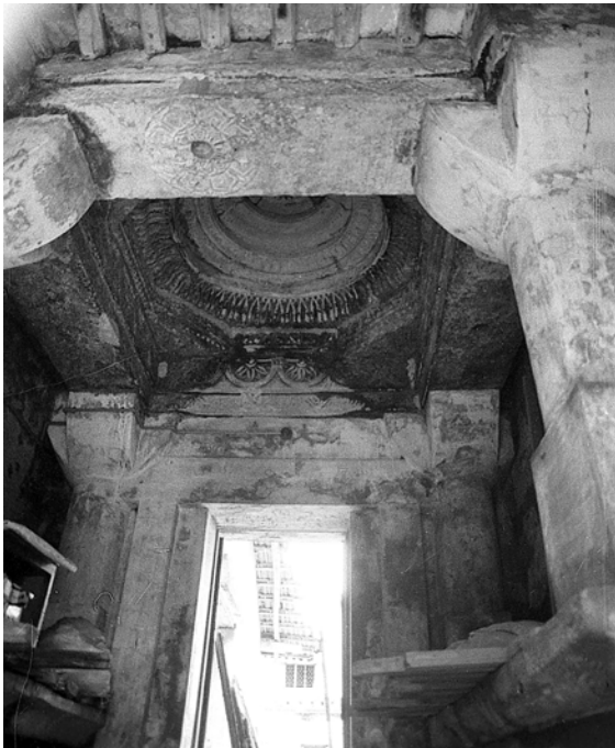
PLATE 4.15 Karao Jāmi', the north entrance to the courtyard, interior of the original domed porch looking north. The columns are plastered over, and the space between them walled up, but the carved details of the lintels and corbelled dome are exposed.
