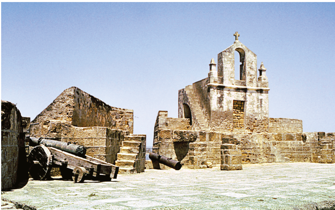
PLATE 3.15 St George's Chapel over St George's Tower (19). The chapel consists of a small chamber topped by an arch which once housed a bell. Most of the chapels on the bastions are closely similar in design, but some are not fully preserved.
