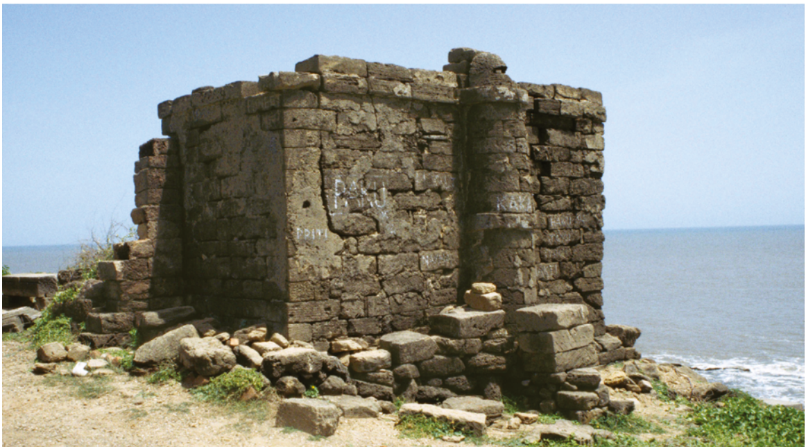
PLATE 6.12 Mosque at Sunset Point, above: view from the east; below: from the north-west, showing the surviving northern and western walls and the projection of the mihrāb .
