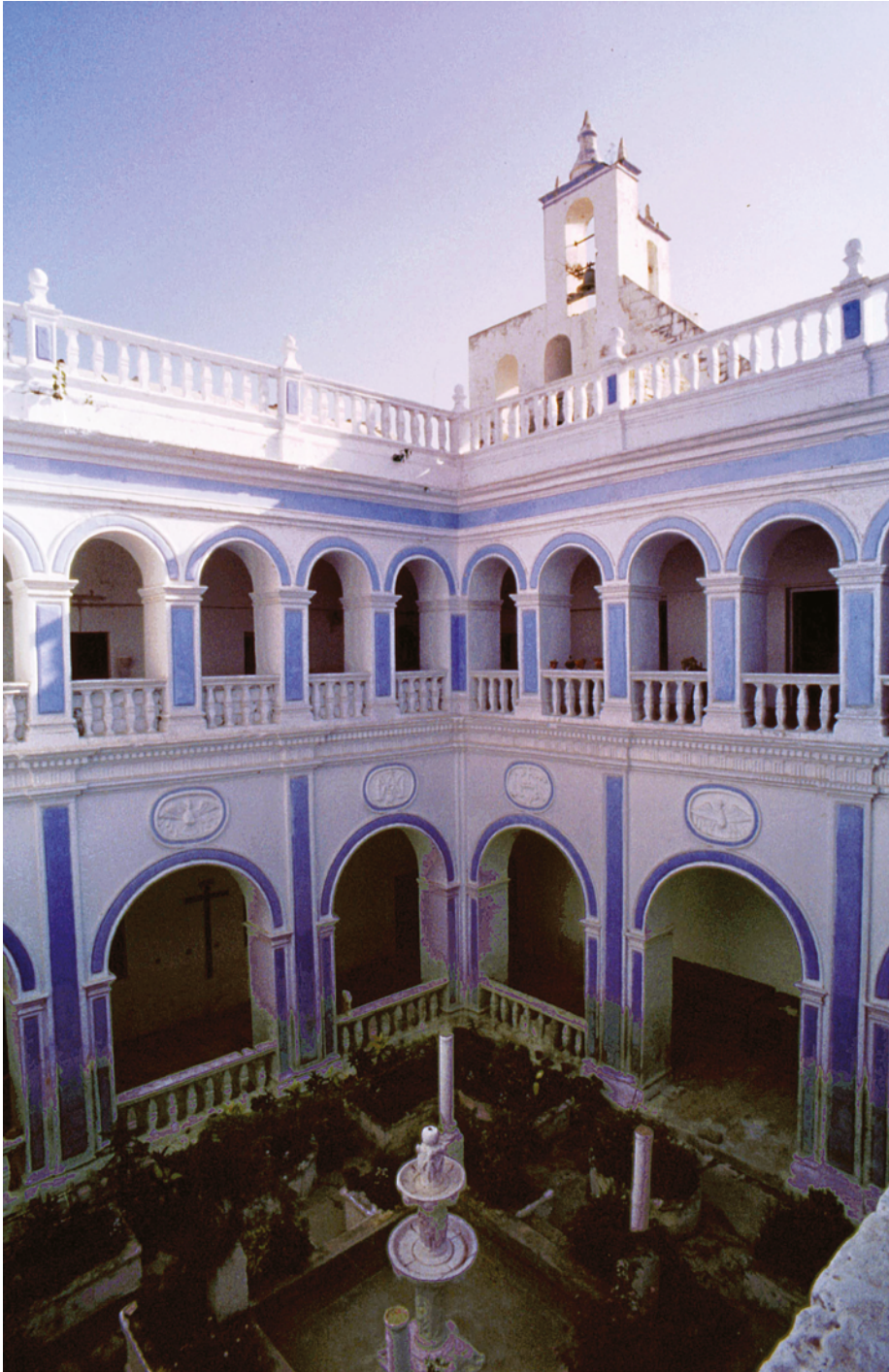
PLATE 4.60 St Paul's Church and Seminary, cloister seen from the north-east. The vaults of the rooms at the ground floor create ceilings higher than those of the upper level. This is reflected in the proportions of the two levels of the cloister with three tall arches at each side below balanced by six smaller arches at the upper level and a fairly high parapet surmounted with balustrades around the roof. The structure on the roof housing the bell and the parapets of the flight of steps to its right can also be seen.
