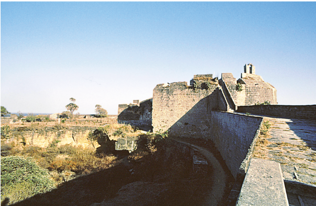
PLATE 3.14 Western fortification walls of 1534–35 looking south-east with the quarry on the left and the Knight's Tower (11) on the right. The tower stands considerably higher than the wall and is reached by flight of steps with the ruins of what seems to have been a chapel at the top. St James's Tower (13) is in the background.
