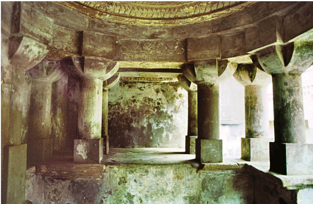
PLATE 4.18 Karao Jāmi', eastern entrance canopy looking north. The original re-assembled carved stone is plastered over, except the soffit of the corbelled dome, of which the lowest course appears in this photograph.
