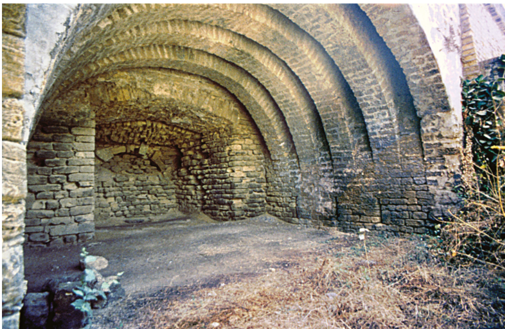
PLATE 3.11 St Philip's bulwark (12). Chamber built into the tower at the level of banquette of the wall.
