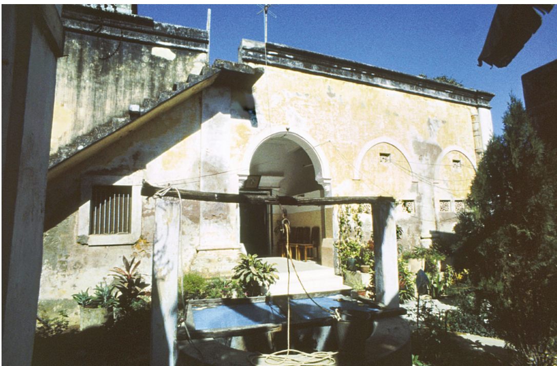
PLATE 5.5 Former fire temple, view of the east side of the building showing the arches of the eastern portico, two of which are now blocked up. The arch at the north side of the portico, not seen in this photograph, is also blocked converting the portico to a chamber. Cantilevered stone steps lead to the roof. In the foreground is the well with a bucket for drawing the water with a rope and a pulley.
