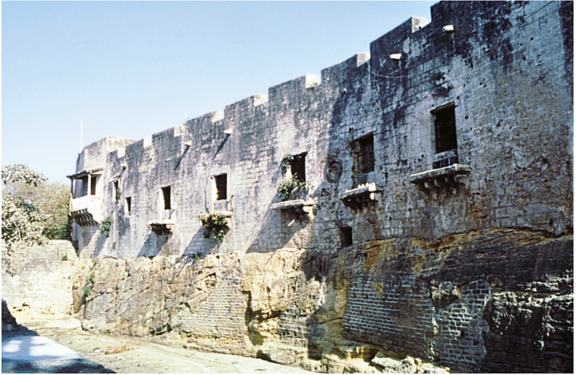
PLATE 3.30 The Old Governors' Residence (6) external façade seen from the causeway (i) looking south-east. Most of the features are original, including the stone water-spouts below the battlements and the balconies in front of the windows, but the parapets of all the balconies have been lost and that of the large balcony of the main hall at the far end has been reconstructed.
