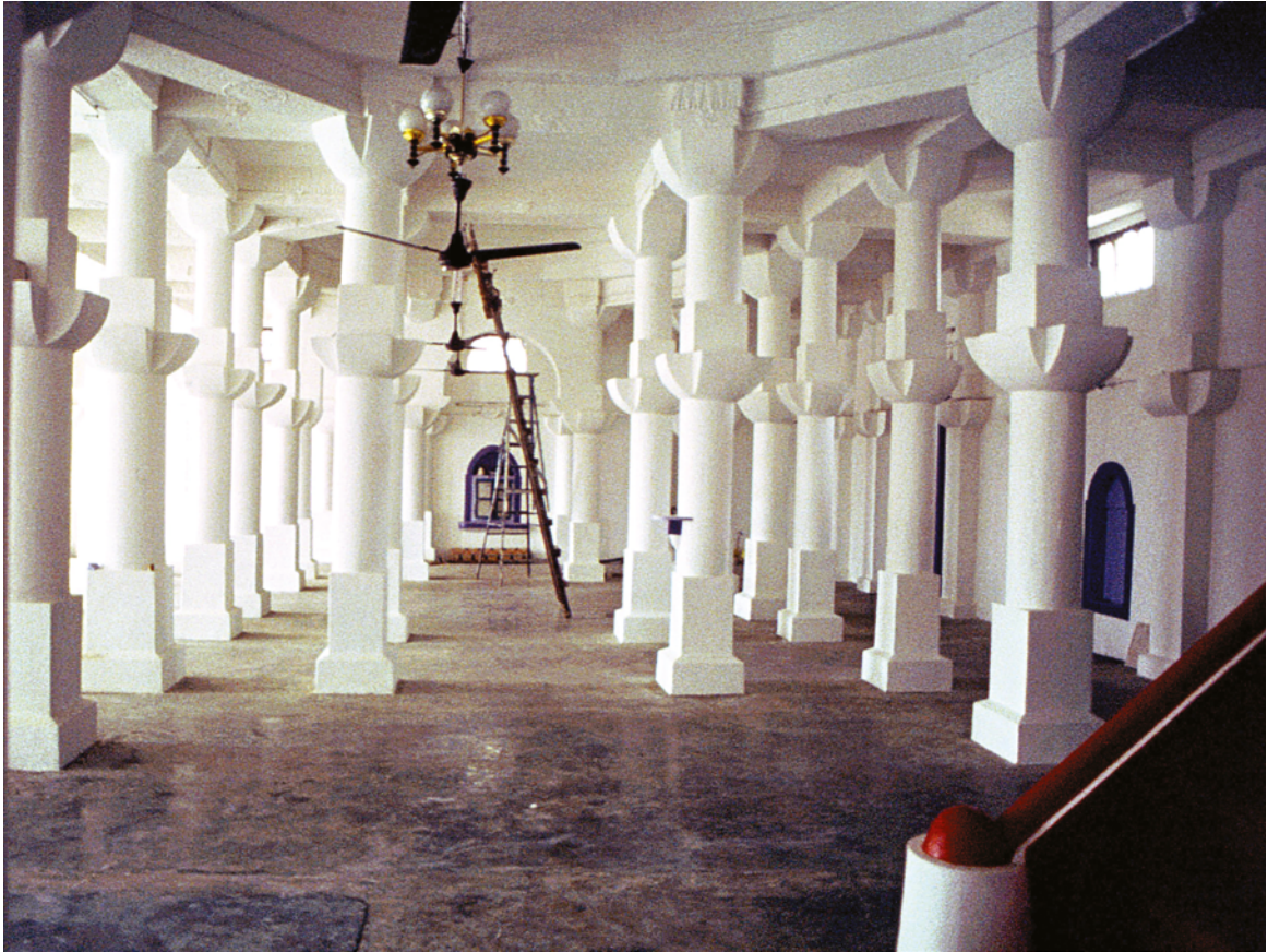
PLATE 1.2 The Karao Jāmi' Mosque, an early-fourteenth-century structure in the heart of the town of Diu. The columns and other structural elements are reused spoil of earlier Hindu and Jain temples, plastered over to obscure the original carvings. The survival of the building under the Portuguese, known for their destruction of Muslim edifices, may seem surprising, but the relationship of the Portuguese with the Sultanate of Gujarat differed from that in their other Portuguese settlements.
