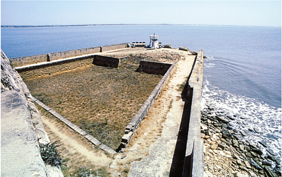
PLATE 3.25 The Indian style reservoir (d) in the fortified breastwork (16) at the eastern tip of the fort, view from the top of St Lucy's bastion (15) looking east. The lighthouse (e) behind the steps of the reservoir at the north-eastern edge of the breastwork is modern.
