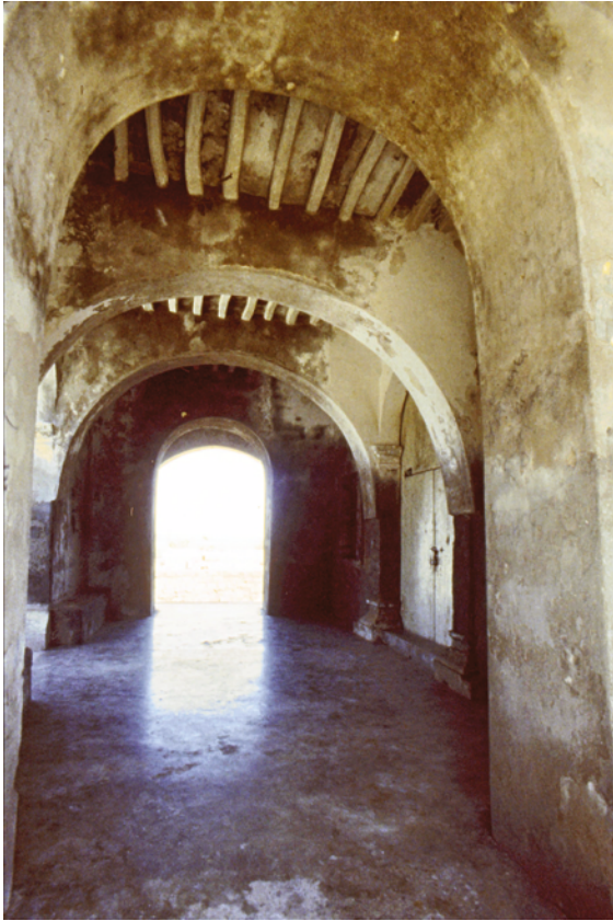
PLATE 6.37 Vanakbara, Church of Our Lady of Mercy, veranda, interior looking north, with the entrance to the church at the right. The ceiling is constructed with wooden rafters, not all straight pieces and only roughly planed.
