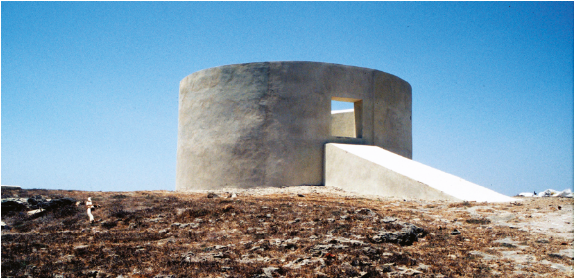
PLATE 5.14 South Tower, general view from the south-east.
