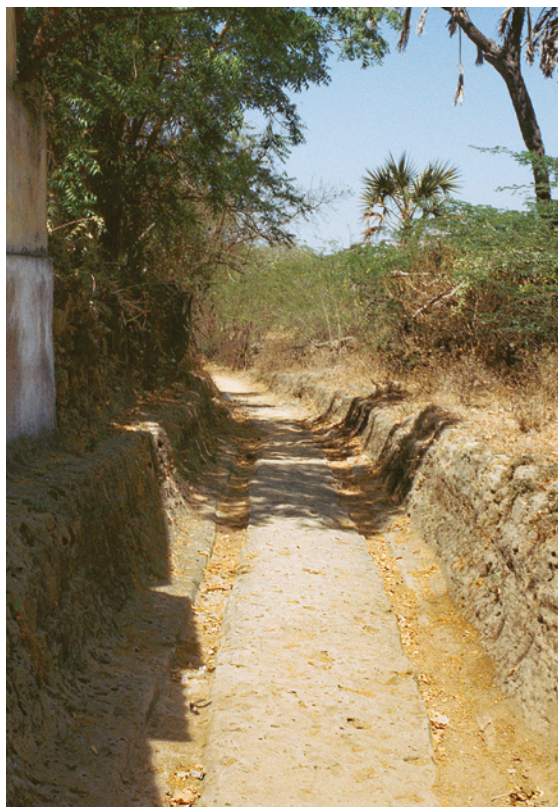
PLATE 6.18 Mediaeval road from the town of Diu to Fudam and the west of the island, carved into the rock to keep it level, with cart tracks visible on the surface. Farming has erased traces of the road where it was laid on earth.
