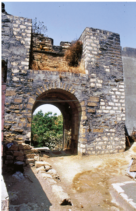
PLATE 4.30 Western town wall, southern postern gate (m) from the town side. The wide and deep niche over the entrance might have been vaulted and used originally as an observation post. Through the opening the overgrown moat can be seen where once a drawbridge stood.
