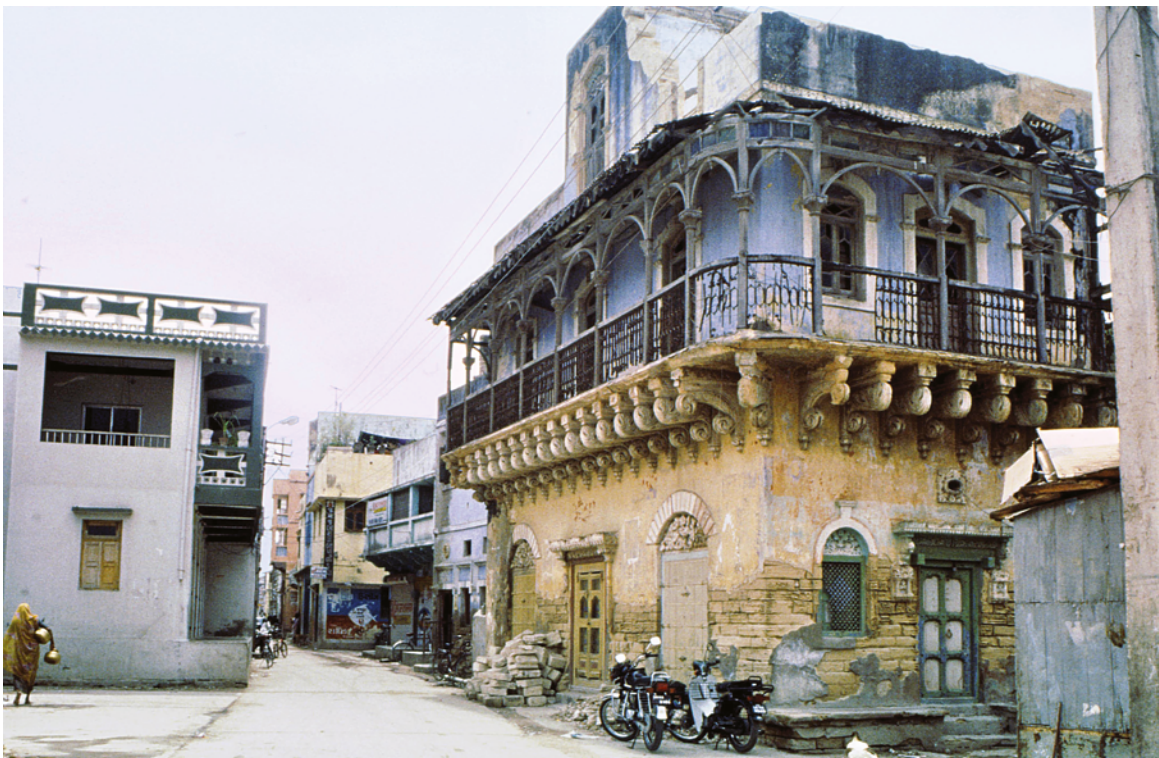
PLATE 4.69 Ghoghla, traditional and modern residential buildings on the street leading from the north-east gate, view looking south-west. The old house on the right combines Portuguese colonial influences with Gujarati features such as the stone brackets supporting the balcony, and the old carved doors, which were falling out of favour with a preference for rebuilding plain practical houses in concrete. More appreciation is now being felt for the old styles and craftsmanship.
