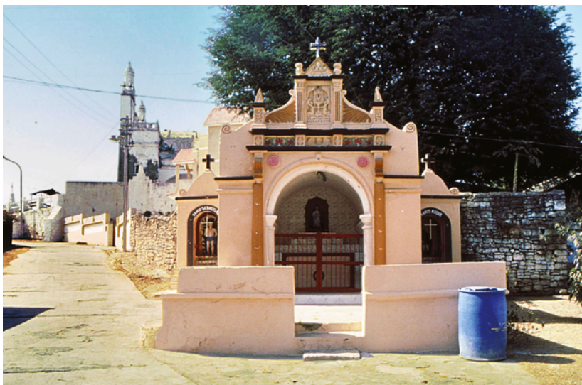
PLATE 4.66 Shrine of Our Lady of the Immaculate Conception (p), general view from north. Above the arch of the main shrine the string course with blocks decorated with diamond patterns can be seen and above that is the inscribed panel carved with two angels holding the tabernacle. On the pediment above the bust of Jesus emerging from the clouds can just be identified. Two small shrines attached to the main shrine are that of St Sebastian at the east (left) and that of St Roque at the west (right).
