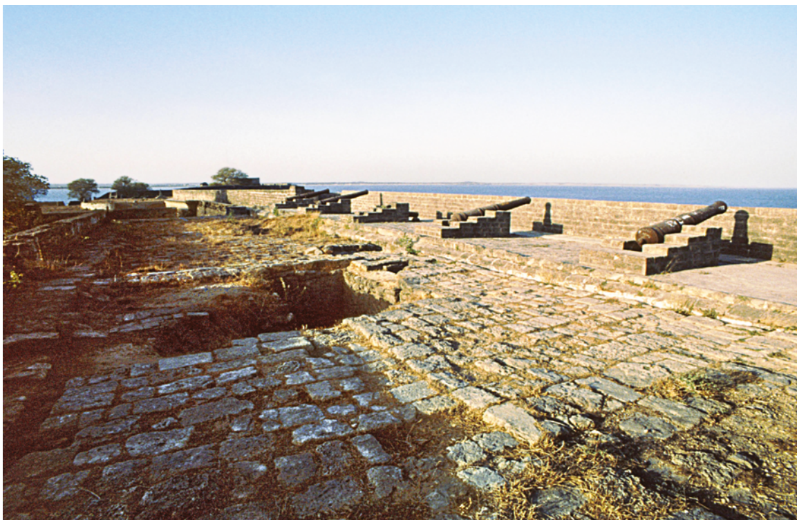
PLATE 3.21 The reservoir (25) attached to Chato's Tower (14). The tank is partly constructed above ground, up to the level of the banquettes of the south-east side of the fort. View from the roof looking north-east showing the banquettes on the right and the rainwater channels on the left. The fixed supports for cannon and the paving of the surface of the banquettes are modern.
