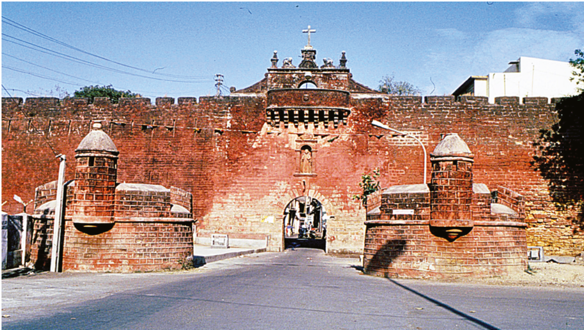
PLATE 4.26 Porta da Terra or the Inland Gate (no. 58) from the fields outside the town looking east. The two towers in the foreground originally flanked a drawbridge which has been removed and, in its place, a solid foundation constructed for the road leading to the gate.
