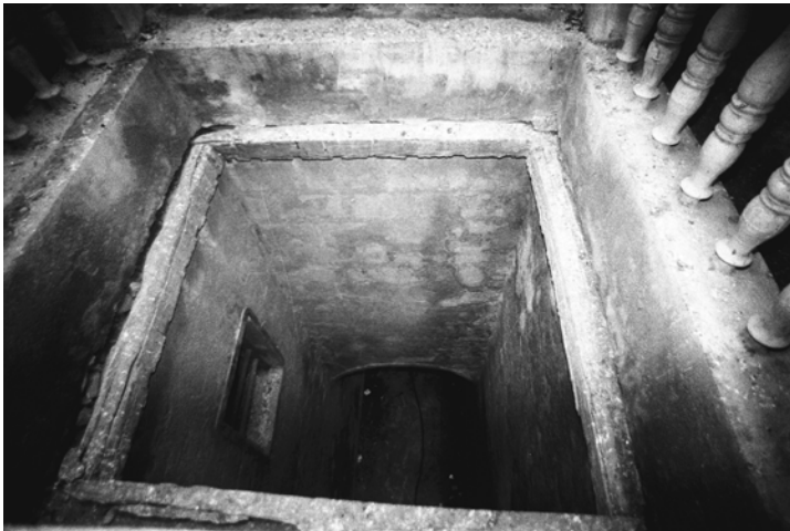
PLATE 3.52 Forte do Mar, chamber below the roof looking down the shaft in the middle of the floor to the corridor which connects the two courts. The shaft is wide enough for cannon and other equipment to be lifted up to the chamber and to the roof of the keep. The window to the left provides meagre light to the stairs from the corridor to the chamber.
