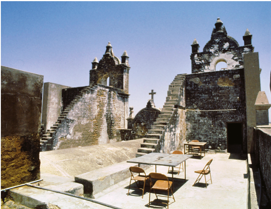
PLATE 6.24 Church of Our Lady of Remedies, view of the roof looking north-east towards the back of the two walls with arched openings for hanging bells, accessed by two flights of steps. The walls give the effect of bell-towers on the eastern façade (Plate 6.22, right). The exterior of the vault of the nave can also be seen between the stairs.
