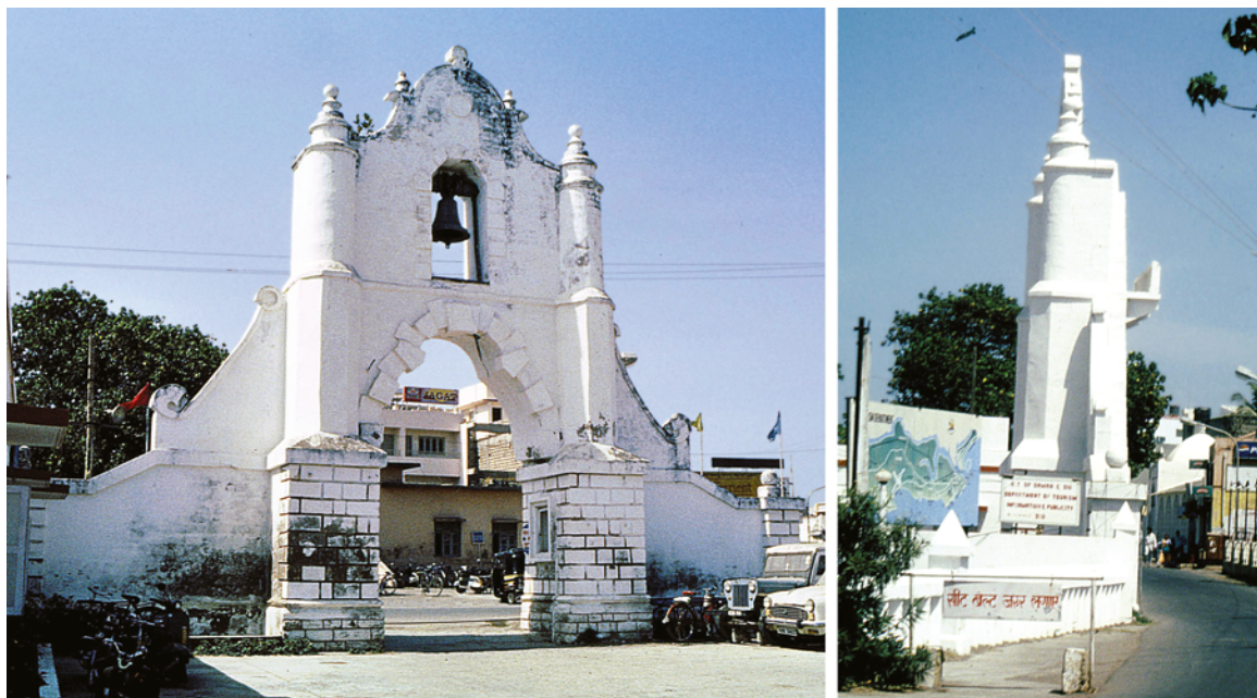
PLATE 4.34 Porta do Mar , left: northern façade and right: view from the west. The niche which once had an icon can be seen in the right pier of the arch.
