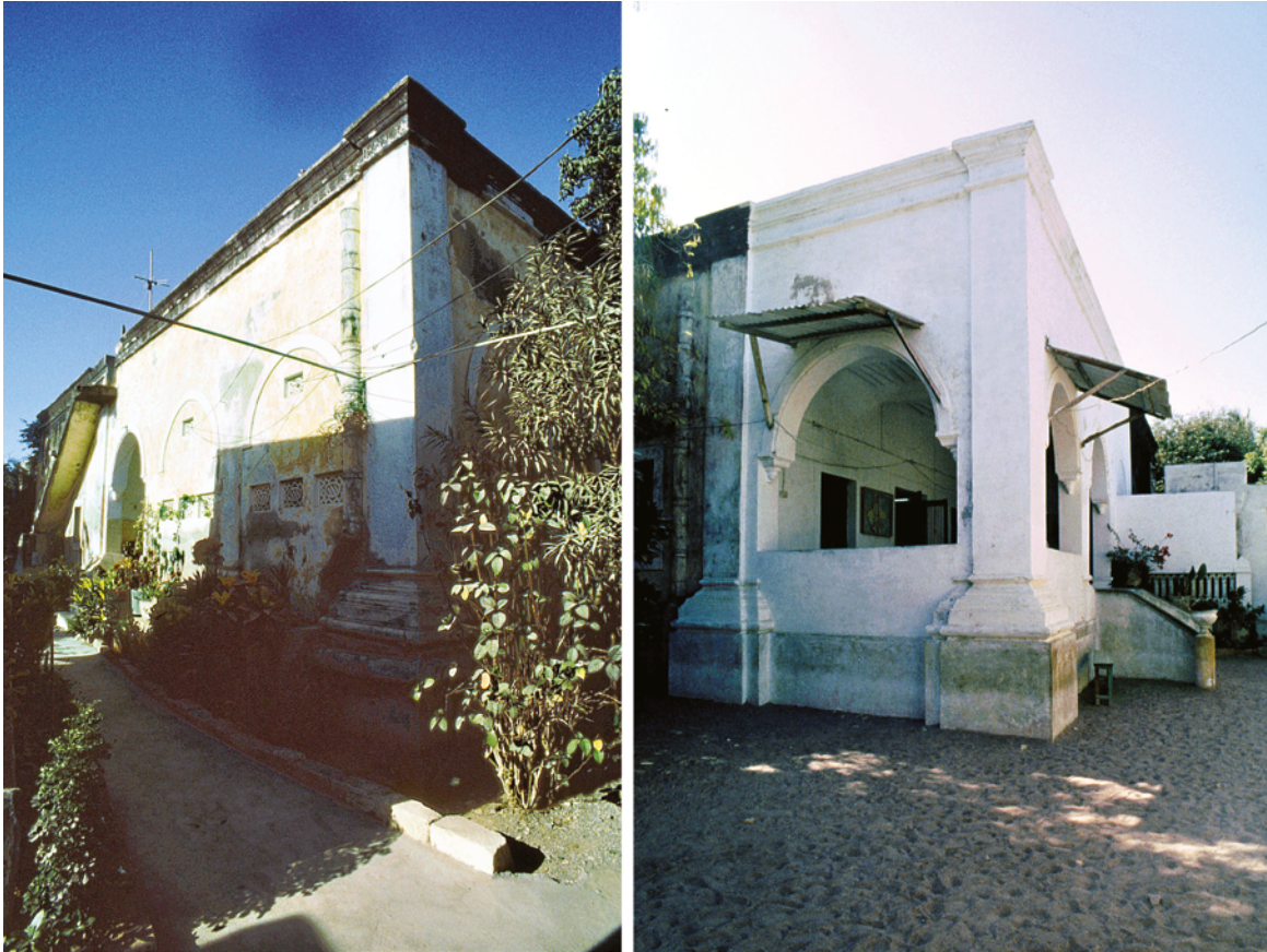
PLATE 5.1 Diu town, the Zoroastrian fire temple, now St Anne's Convent and School. Left: view from north-east showing two of the walled-up arches of the loggia style portico. Right: view from north-west, with the portico left in its original condition. The corner pilasters and raised podium, as well as cornices decorated with cyma recta moulding can also be seen. The steps to the portico at the far right are original.
