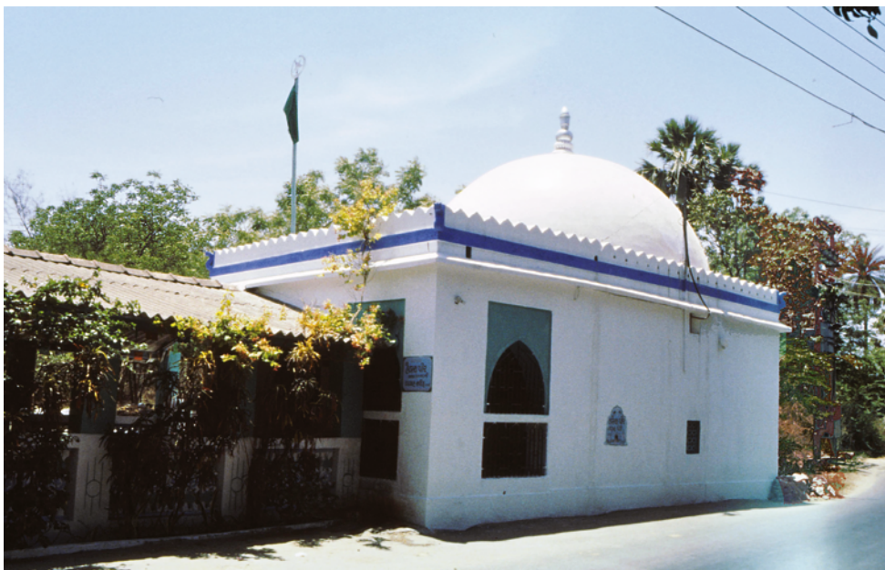
PLATE 6.29 The shrine of Pīr Ḥabash Bābā, view from north-east. The veranda appears to be later in date. It is not keyed to the domed chamber, indicated by a line on the exterior wall, and its crenulations differ from those of the domed chamber.
