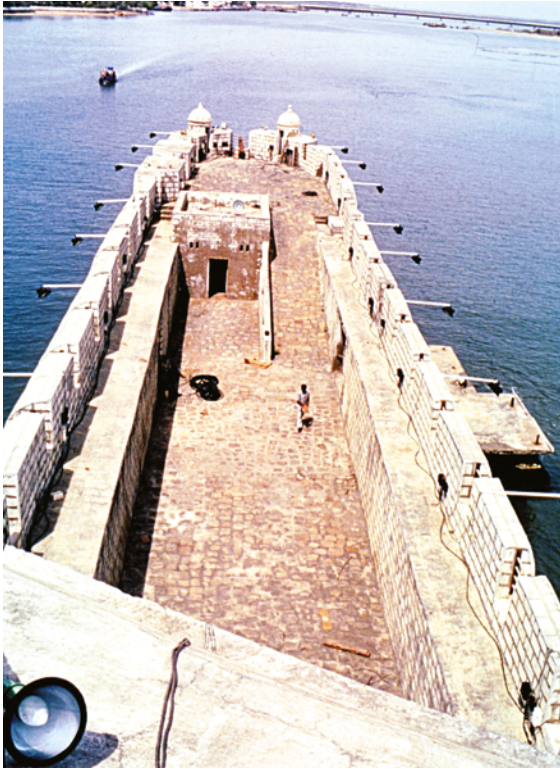
PLATE 3.47 Forte do Mar, north-western courtyard seen from an aperture in the upper chamber of the keep. While the wide walks behind the battlements are for guards to circulate, they are not wide enough for placing cannon. The cannon emplacements were restricted to the main keep and the two ends of the building.
