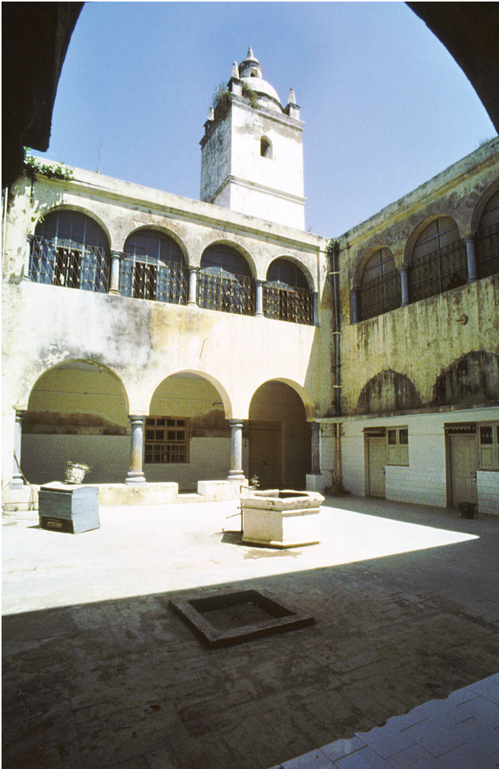
PLATE 4.54 St Francis's Monastery, view of the cloister looking north. The arches of the east side of the cloister have been walled up, and the space is made into a room, but under the modern walls the original structure is intact and the arches can still be seen. The octagonal well-head in the centre of the courtyard opens to a cistern.
