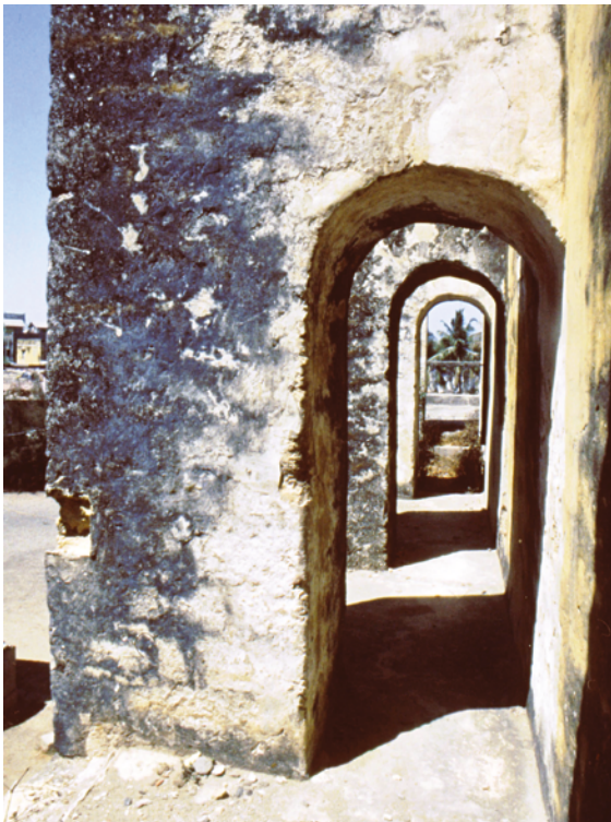
PLATE 6.41 Vanakbara, Church of Our Lady of Mercy, the roofless passage at the upper level, south side, giving access to the western gallery and to the roof of the veranda, view from east end looking west.
