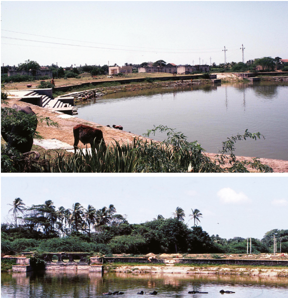
PLATE 6.20 Veraval, Bhal ka Talão . Above: view towards north-west, showing the ghats around the reservoir, the western ramps at the top right and modern stairs built in place of the southern ramp at the left. Below: looking north towards the three sluice gates.
