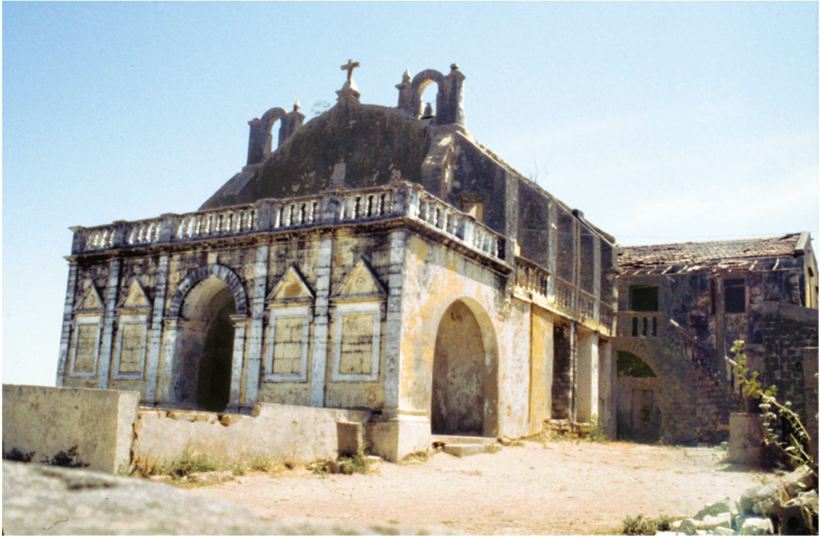
PLATE 6.36 Vanakbara, the Church of Our Lady of Mercy (26), view from the south-west. On the right are the stairs to the chapter house and open walkway which passes through arched openings in the buttresses, giving access to the gallery over the west end of the nave as well as to the terrace over the porch. The door below the stairs opens to the ante-chamber of the sacristy.
