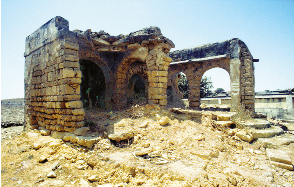
PLATE 6.27 Fudam, old building in the cremation grounds, general view from south-east. The eaves of the patio and part of the fallen roof of the southern wing can be seen.
