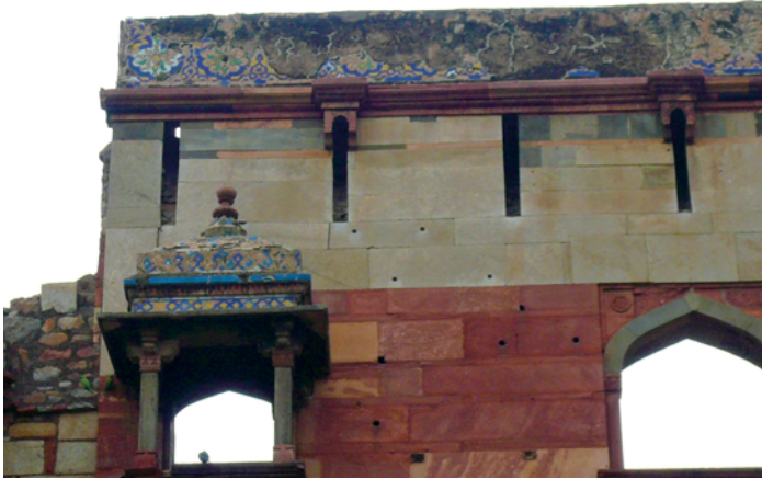
FIGURE 4.35 Bara Darwaza, Purana Qila, 1560s (?), Delhi. Detail of the upper section, with polychrome tile mosaic
