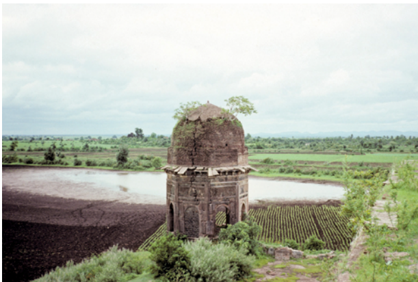
FIGURE 4.91 Malcolm ki Kothi, now-collapsed eastern pavilion PHOTO Y. PORTER, 1989
