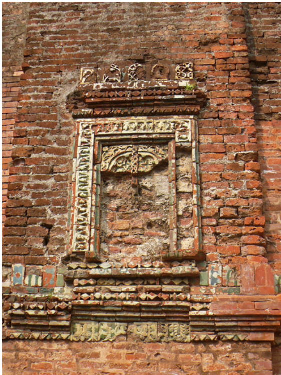
FIGURE 4.49 Chika or Chamkan Building, panel in form of a niche with lamp motif PHOTO Y. PORTER, 2010
