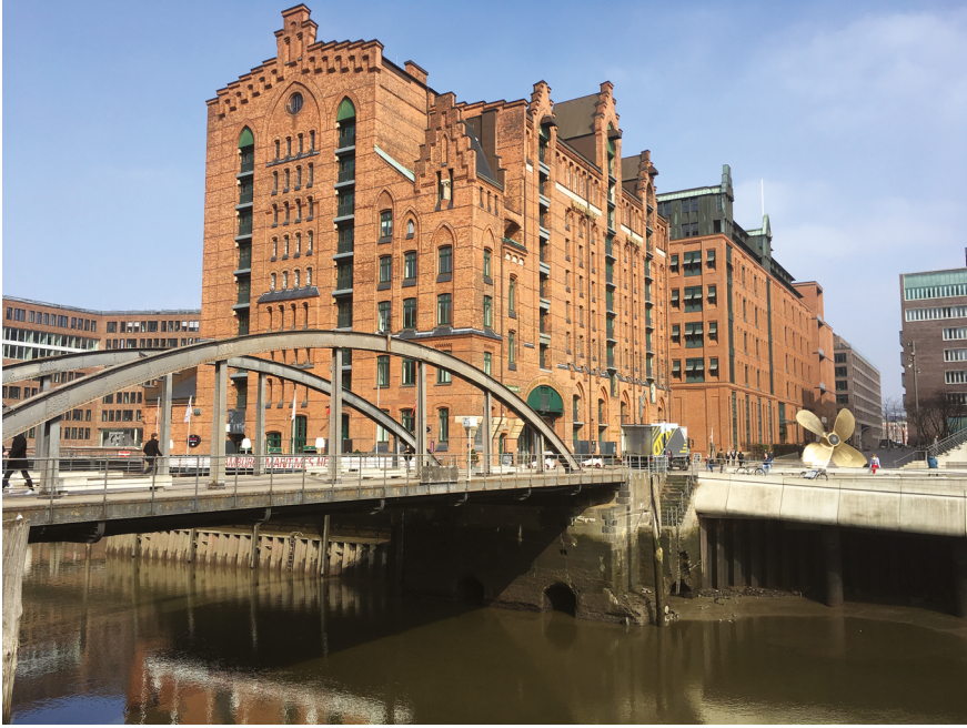
FIGURE 4.1 Historic warehouses and new additions in the Hafencity Hamburg PHOTO: CAROLA HEIN
