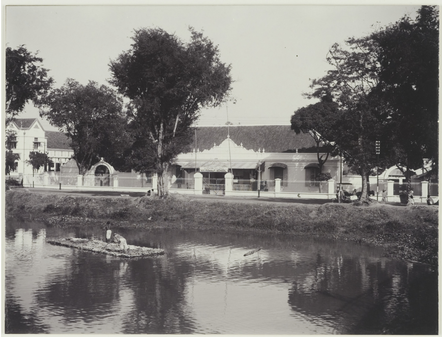
FIGURE 2 Hadramaut School, Surabaya (1924) PHOTO COLLECTION KITLV, LEIDEN, SHELF MARK 2975
