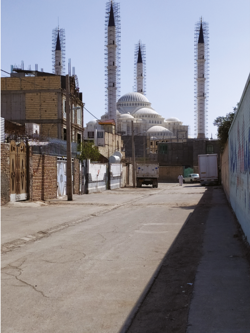
FIGURE 1 Makki Mosque in Zahedan under construction DATE: OCTOBER 2019. PHOTOGRAPHER: SINA HABIBI
