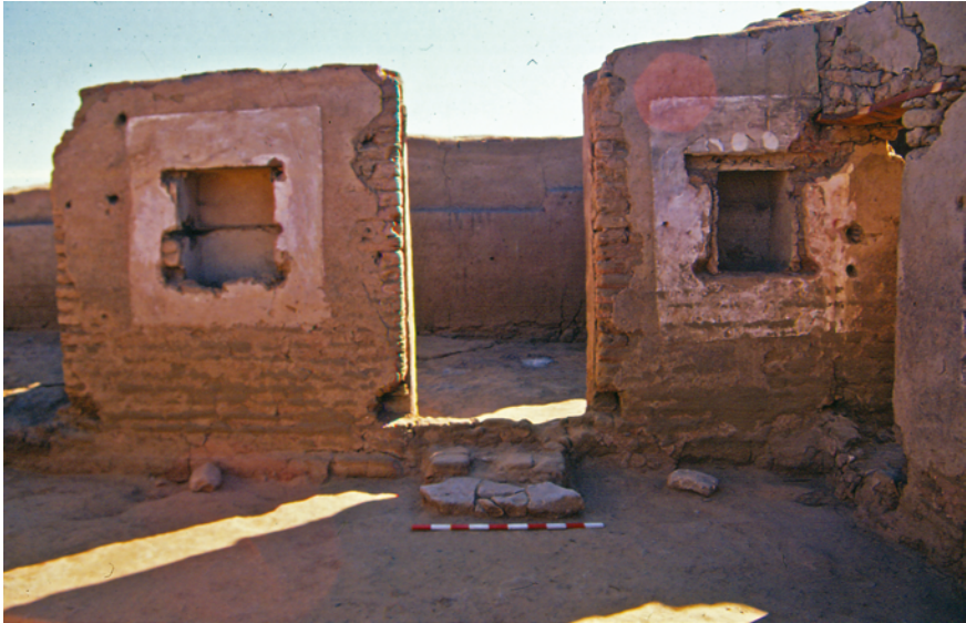
FIGURE 6 The mud-brick walls with plastered niches of House 3 (room 6) COURTESY OF THE DAKHLEH OASIS PROJECT AND COLIN A. HOPE
