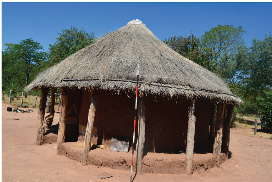
FIGURE 4.1 Cone-on-cylinder type houses
