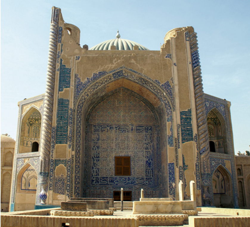
FIGURE 2.4 AKTC mausoleum-mosque restoration with suffah of Parsa'i burials in the foreground
