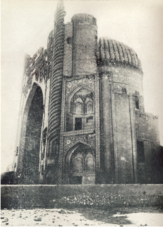
FIGURE 2.20 North wall; note structure projecting from southeast corner of the mausoleum SĀLNĀMAH-I KĀBUL , 1934
