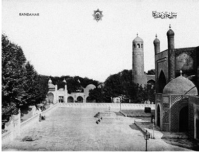
FIGURE 3.19 Riwāqs along north wall and langar-khānah SOUVENIRS D'AFGHANISTAN , 1925
