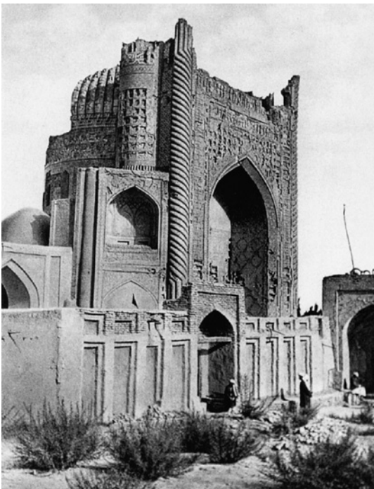
FIGURE 2.23 Southern wall extension enclosing part of the cemetery O. VON NIEDERMAYER, 1916
