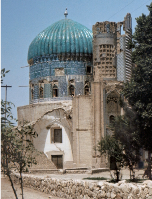
FIGURE 2.28 Post-1956 earthquake showing collapsed section, missing cloister seen from the south DR. GREMLIZA, 1967
