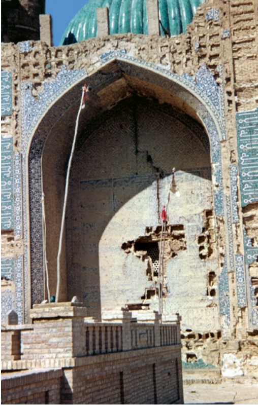
FIGURE 2.7 Grille window begins to show in blind wall of the pīshṭāq H. FRUMKIN, 1954
