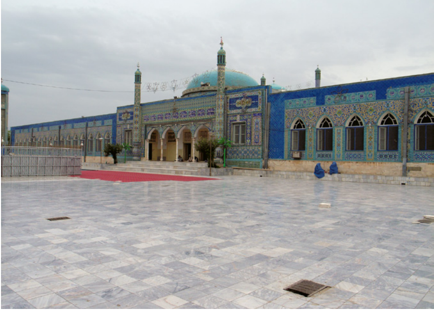
FIGURE 3.33 Paramach Mosque (east façade (back side) as seen from the northeast) enclosing Nazargah Gate (center portion under smaller dome) B. WOODBURN, 2007
