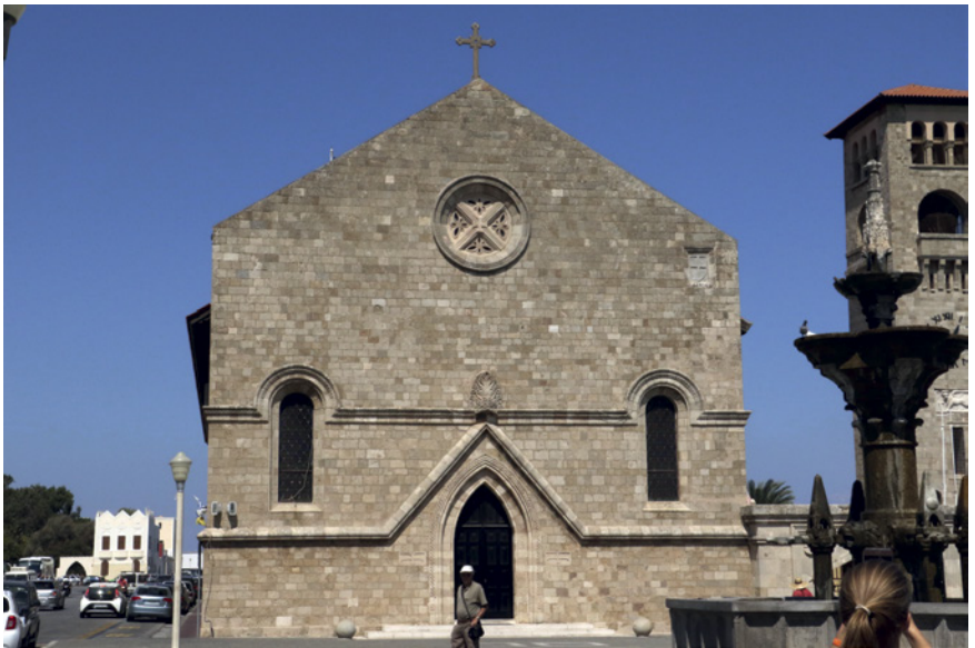
FIGURE 16B The church of the Annunciation, 1924/1925–1929, Mandraki port. View from the west
