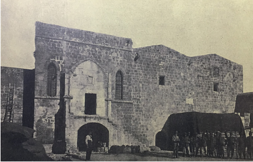
FIGURE 47A The earlier hospital, first half of the 14th century, Rhodes. East facade before the restoration
