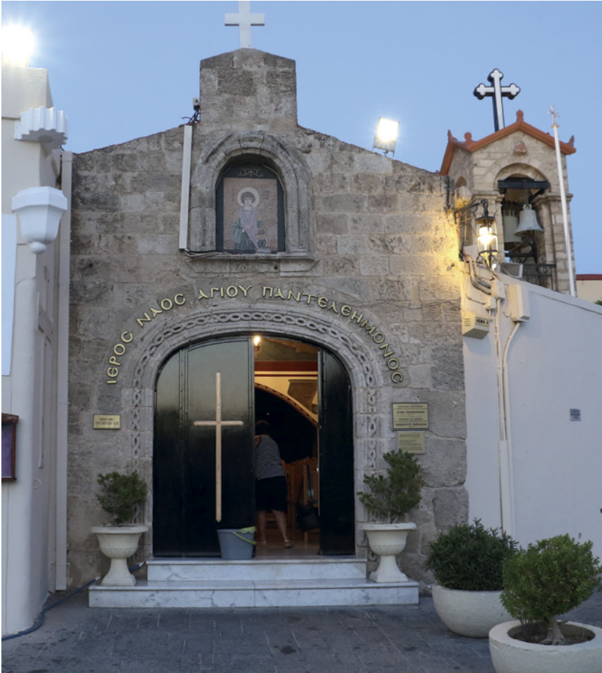
FIGURE 59 St. Pantaleon, west entrance currently
