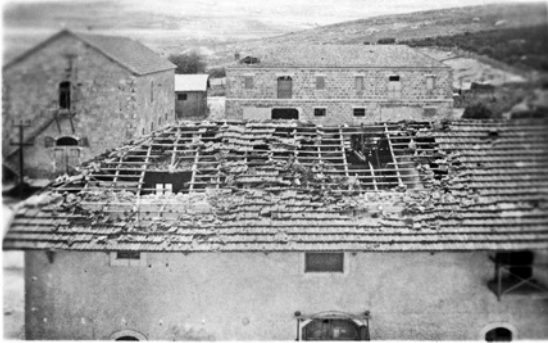
FIGURE 2.2 Damage to Trappist Monastery, Latrun, 1948 AATL/AEBAF
