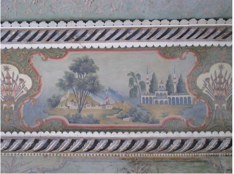
FIGURE 17.33 Bayt 'Abd al-Qādir al-Ġazā'irī, house in the middle of 'Abd al-Qādir's five adjacent houses, room in first floor of the south wing, detail of the ceiling cornice with characteristic mid-nineteenth-century landscape painting PHOTO: ANKE SCHARRAHS, 2011
