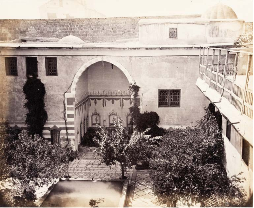
FIGURE 17.18 Bayt Sa'īd al-Quwatli/al-Murādī/ British consulate, 1862, historic photograph of the inner courtyard ( ḡuwwānī ) with īwān and large fountain, view to the south. The room east of the īwān (left of īwān in the photograph) is depicted in Wild's drawing E.3855–1938 (fig. 17.16). This photo documents the layout of the house as Wetzstein might have seen it, before the renewal of around 1870. PHOTO: FRANCIS BEDFORD, 1862, © VICTORIA AND ALBERT MUSEUM
