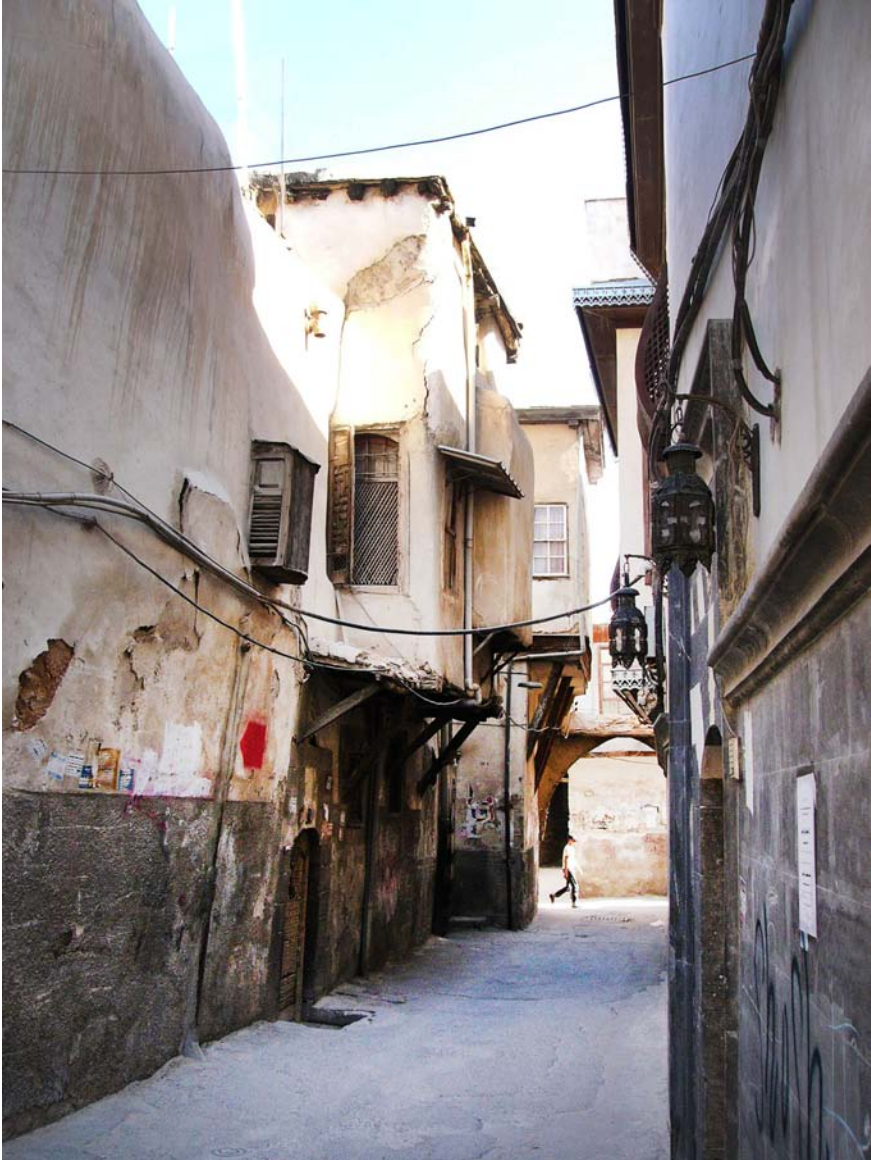
FIGURE 17.1 Old City of Damascus, al-Šahbandar street looking north, with characteristic plain outer walls of traditional houses and overhanging first floor rooms supported by wooden beams. The building on the left side of the street is the house of the merchant family al-Qaziha. The overhanging room in the center of the left wall is the room in which presumably the American consul Miḥā'il Mišāqa was hidden during the 1860s riots PHOTO: ANKE SCHARRAHS, 2008
