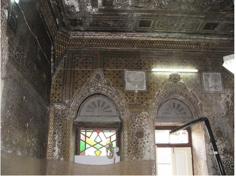
FIGURE 17.35 Bayt 'Abd al-Qādir al-Ġazā'irī PHOTO: ANKE SCHARRAHS, 2011
