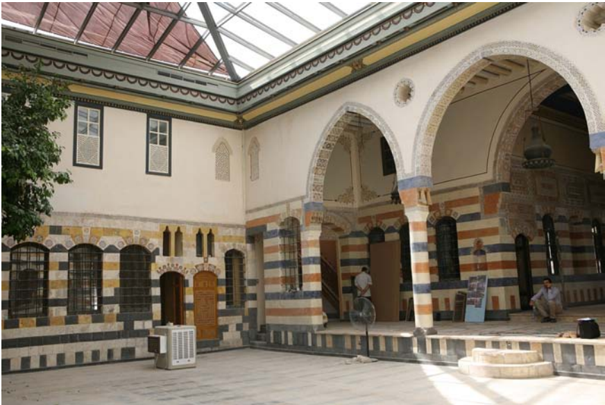
FIGURE 17.14 Courtyard of Bayt Fārḥī/al-Mu'allim, view to the south-west corner PHOTO: ELIZABETH MACAULAY-LEWIS, 2010
