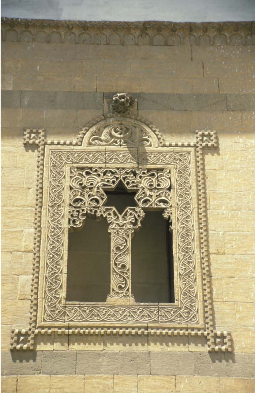
FIGURE 17.9 Bayt Ḥalīd al-ʿAẓm, north-west corner of the northern courtyard, finely cut masonry in the first-floor facade of the “snake salon” PHOTO: STEFAN WEBER, 2006
