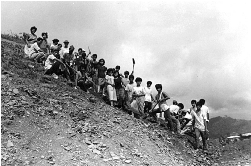
FIGURE 9.8 Communal labor. Improving the Presbyterian Hospital in Durtlang village, 1980. PHOTOGRAPHER UNKNOWN. REPRODUCED BY PERMISSION OF PRESBYTE- RIAN HOSPITAL COLLECTION, AIZAWL, MIZORAM, INDIA
