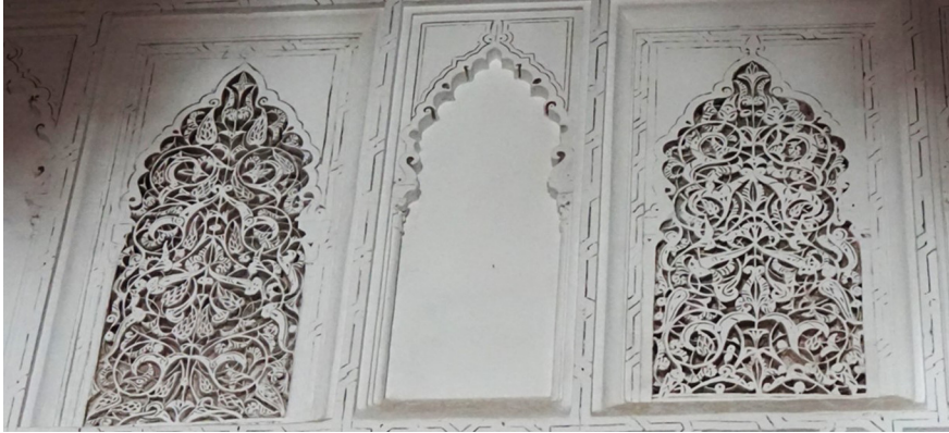
FIGURE 14.8 Detail, Mihrāb façade, Kutubiyya Mosque, Marrakesh AUTHOR'S PHOTO
