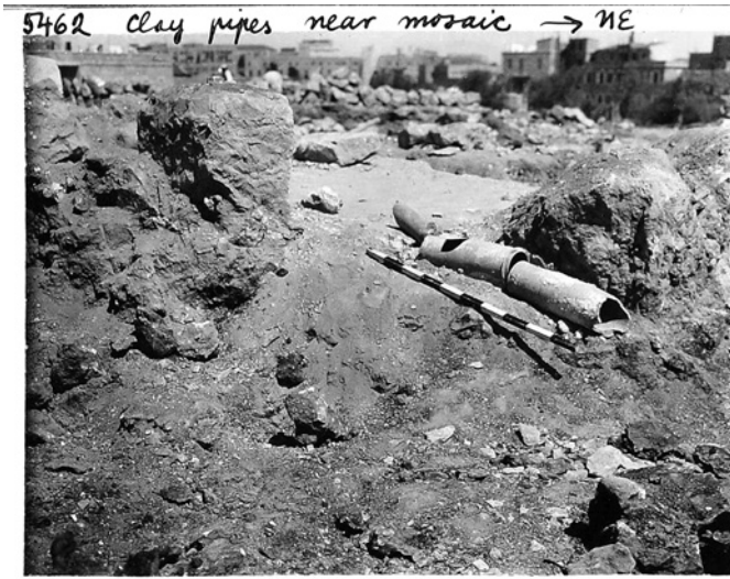
FIGURE 109 YMCA, "Monastery"; clay pipe near mosaic. COURTESY OF ISRAEL ANTIQUITIES AUTHORITY.
