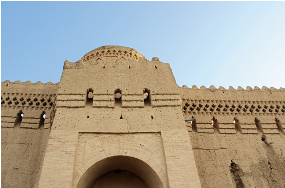
FIGURE 9.6 Machicolations over the gate and on the upper level of the walls, Bāgh Dīyhūk PHOTO: HATEF NAIEMI.
