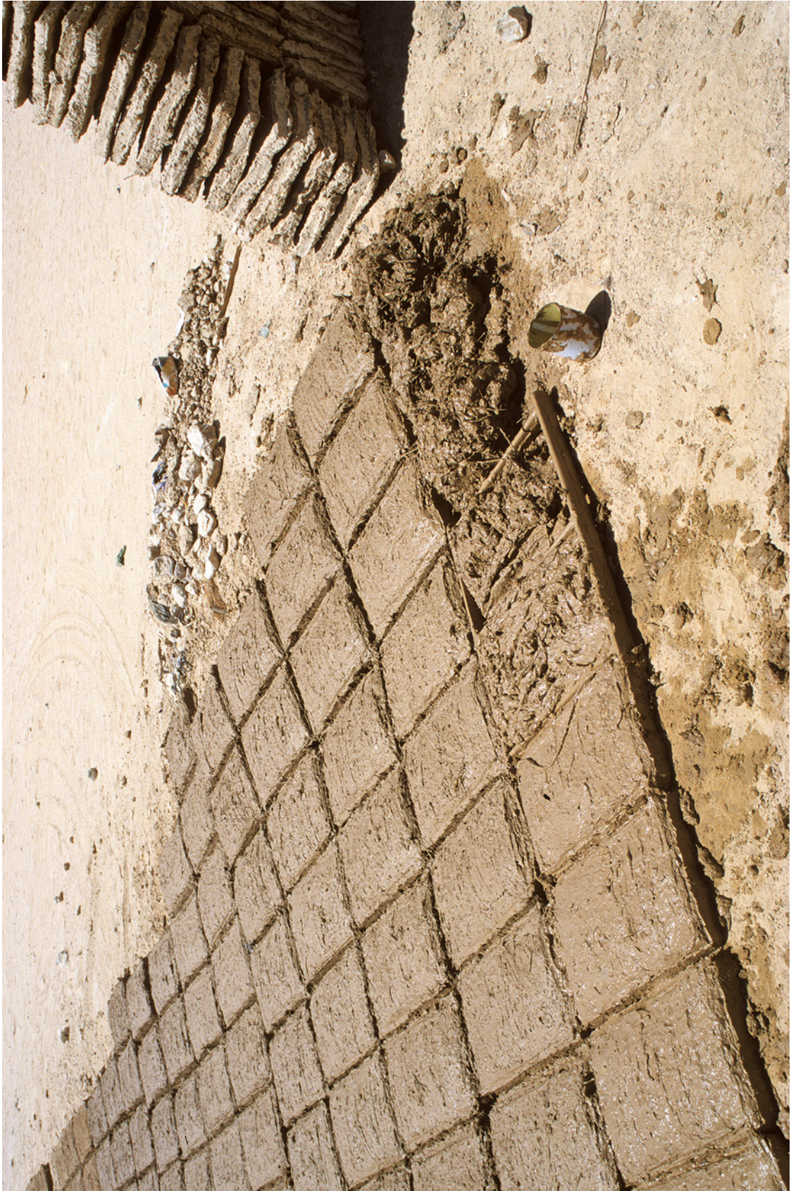
FIGURE 7.11 Bricks are molded flat and occupy a large surface CREDITS: CHRISTIAN DARLES.
