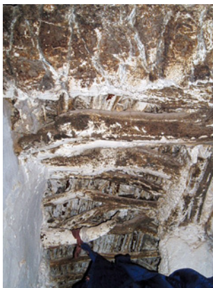
FIGURE 5.13 Ceiling with zizīphus wood in Garrāra, 2009 CREDITS: CHEKHAB-ABUDAYA.
