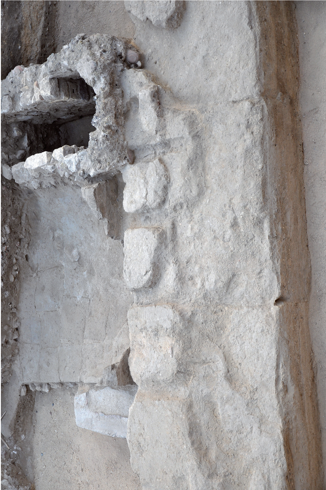
FIGURE 6.7 Photography of a detail of the rammed-earth wall CREDITS: PRADINES.
