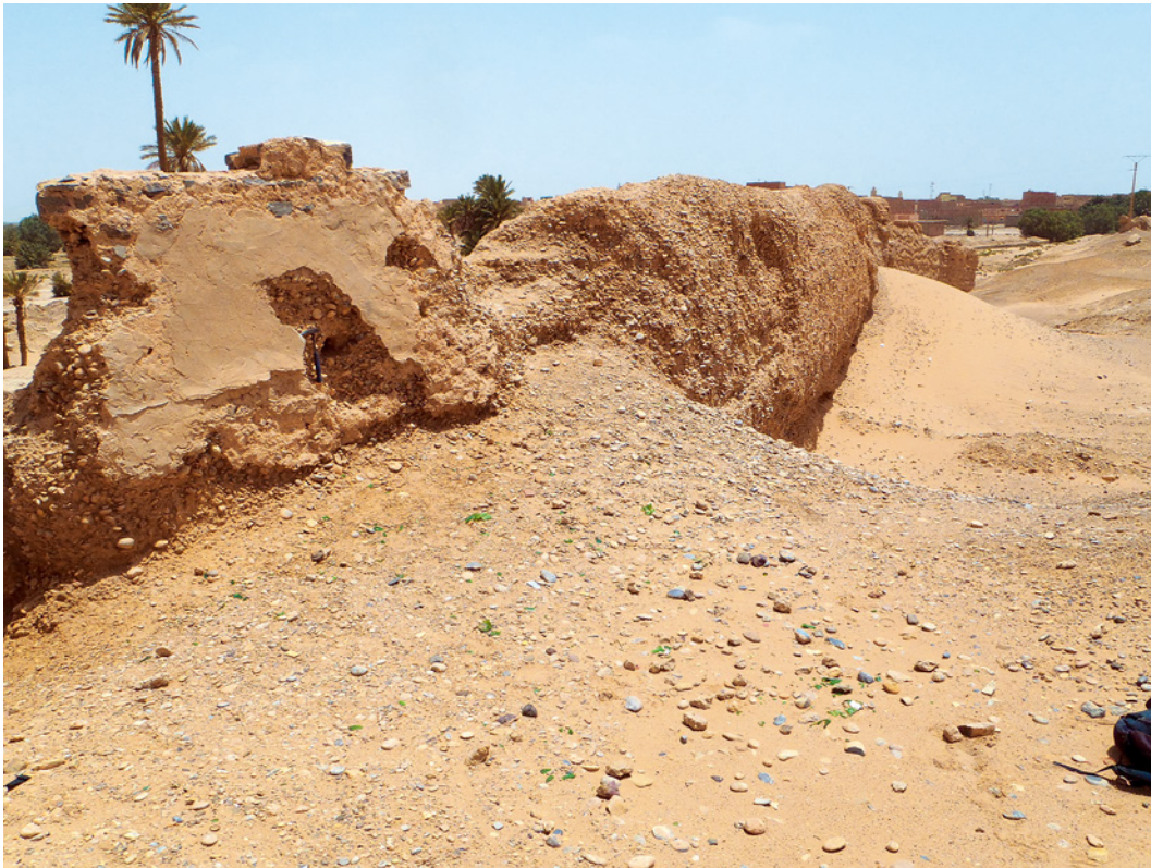
FIGURE 3.8 Photo of the north periphery wall (section 2 in this article; the schist top and the plaster cladding may be recent).
