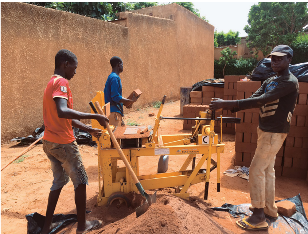
FIGURE 12.2 Compressed earth block production PHOTO CREDIT: MARIAM KAMARA.
