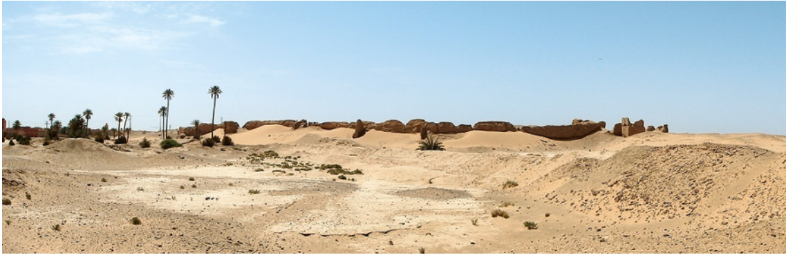
FIGURE 3.7 Panoramic photo facing south, of the north periphery wall (section 2 in this article, dating to the 12th–13th century).
