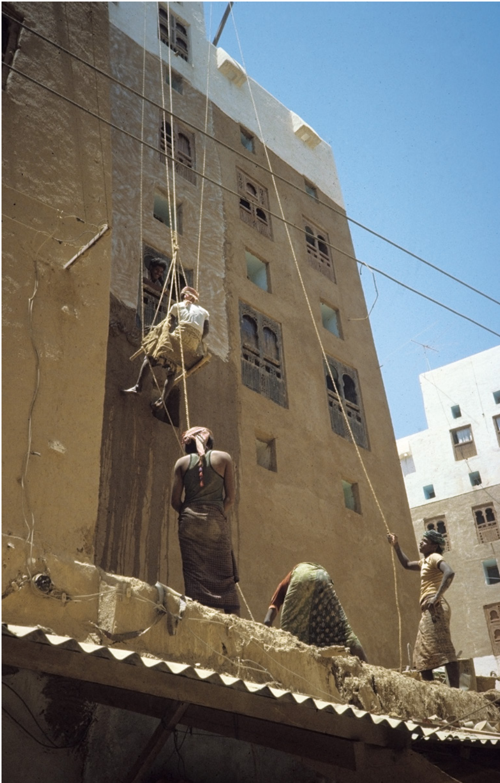
FIGURE 7.16 Plastering work of the façade of the tower houses CREDITS: CHRISTIAN DARLES.
