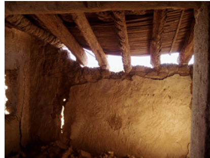
FIGURE 5.8 Use of date palms for the ceiling, Tammāsīn, 2009 CREDITS: CHEKHAB-ABUDAYA.
