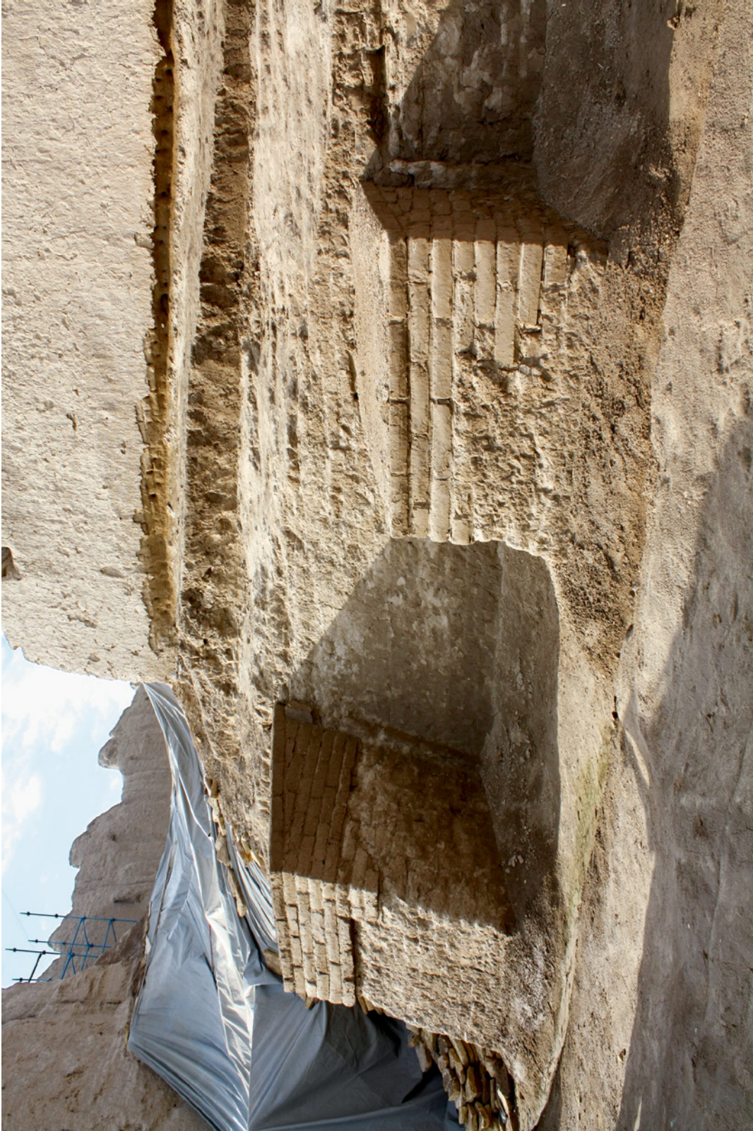
FIGURE 10.2 The lower glacis of the Great Kyz Kala at Merv, showing mudbrick bastions recently excavated by the State Historical Cultural Park Ancient Merv. Note the upper layers are new bricks after conservation
