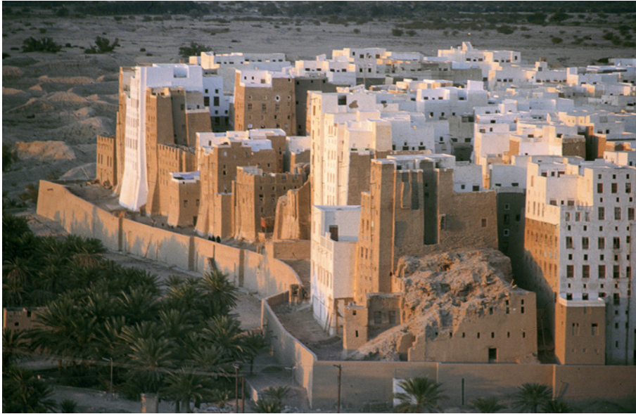
FIGURE 7.14 View of the southwest corner of the City of Shibam with a new destroyed house and the curtain wall CREDITS: CHRISTIAN DARLES.
