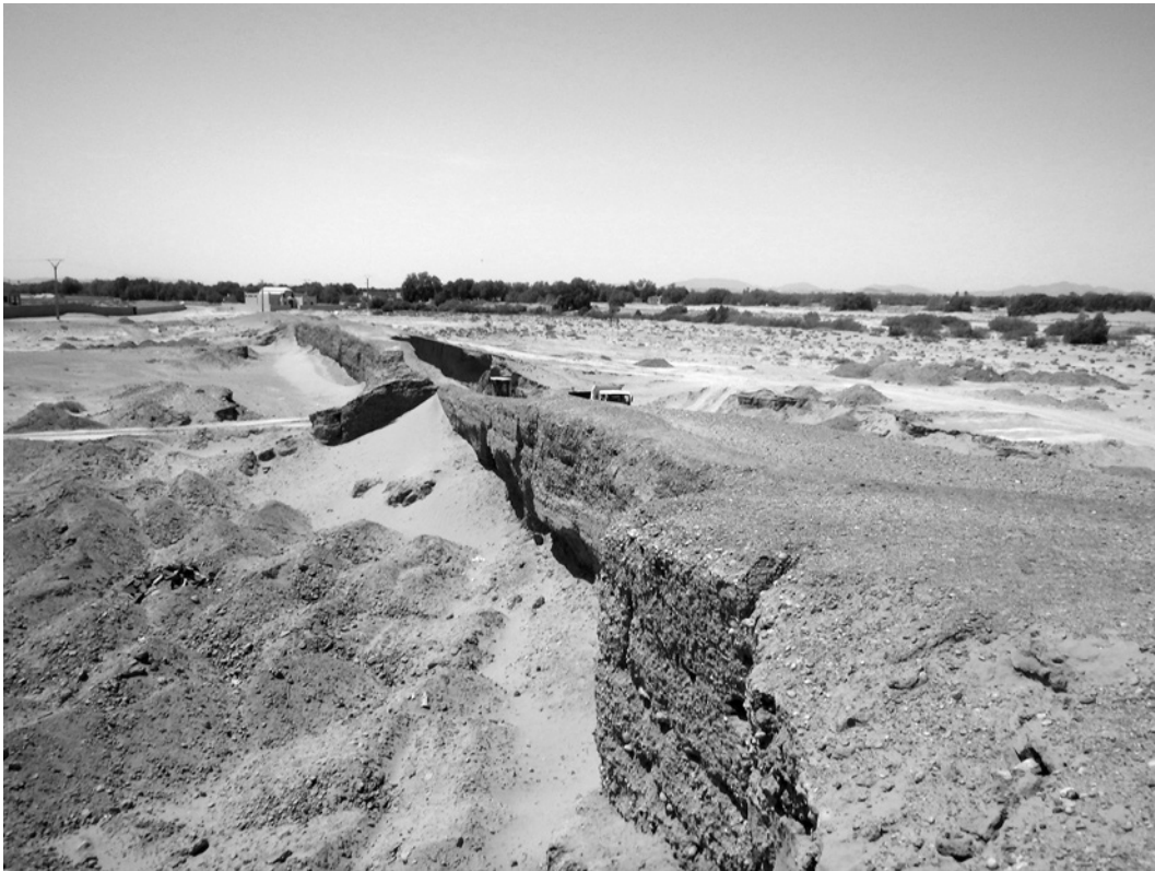
FIGURE 3.5 10th Century periphery wall (section 1 in this article; picture facing south, including a square tower in the foreground, and a truck and backhoe collecting sand in the background). PHOTO: ROMAIN MENSAN 2014.
