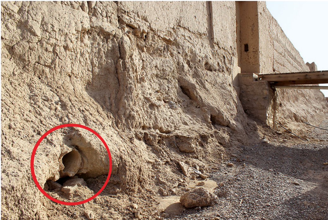
FIGURE 9.17 The earthen tubes were probably used to lead the water of the surrounding moat to the cistern's reservoir; saryazd.
