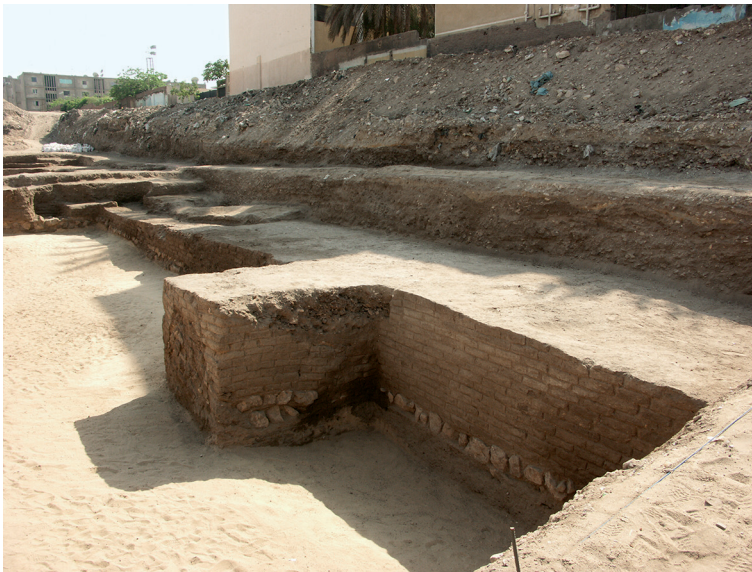
FIGURE 6.21 Photography of a detail of Badr al-Gamali's mud brick wall, beside Bab al-Gedid CREDITS: PRADINES.
