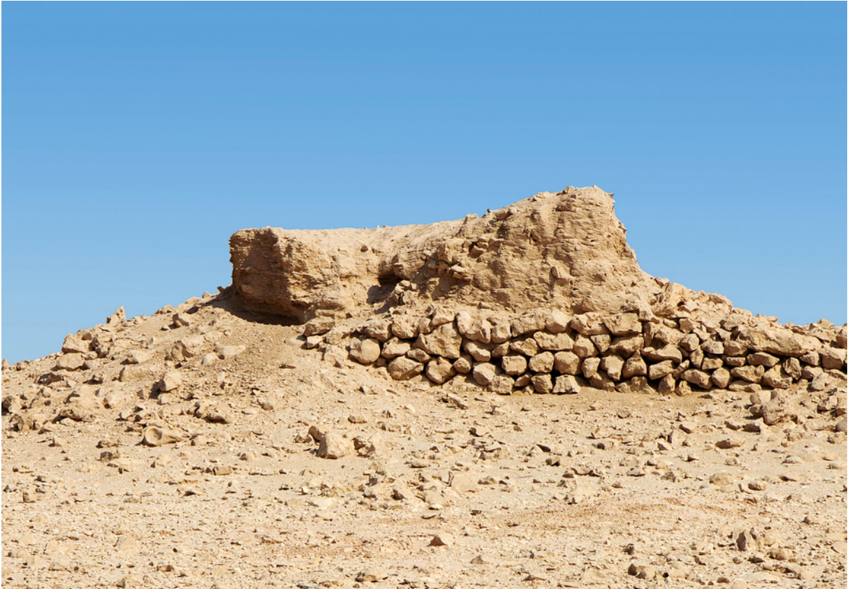
FIGURE 8.15 Qal'at Shuwail: rammed or traditional wet loam wall remains. PHOTO: A. PANTOS, QIAH/UNIVERSITY OF COPENHAGEN.
