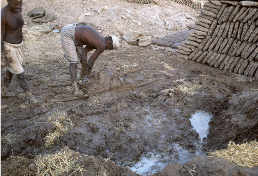
FIGURE 7.9 Earth is mixed with straw CREDITS: CHRISTIAN DARLES.
