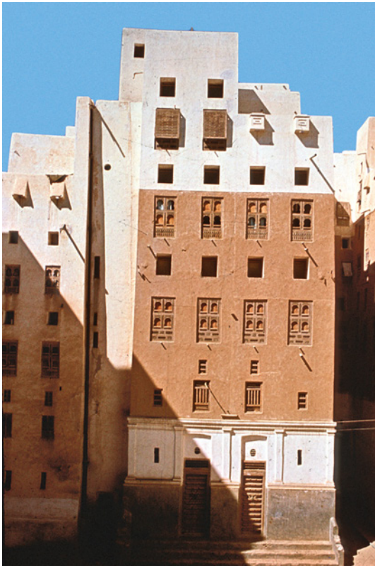
FIGURE 7.5 Tower house of a rich family in Shibam CREDITS: CHRISTIAN DARLES.
