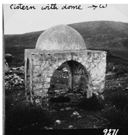
Fig. P27. Cistern before repairs.
