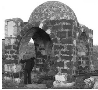
Fig. P28. Cistern after repair.
