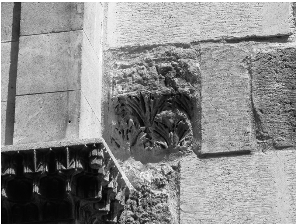
FIGURE 3.3 Late antique pilaster capital reused in the medieval wall of the Great Mosque of the Umayyads, Aleppo AUTHOR'S PHOTO.
