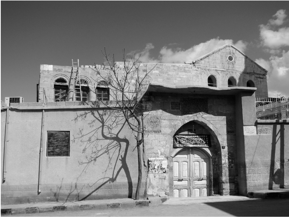
FIGURE 7.4 Exterior of the mosque of al-Qara, a former church converted in the thirteenth century AUTHOR'S PHOTO
