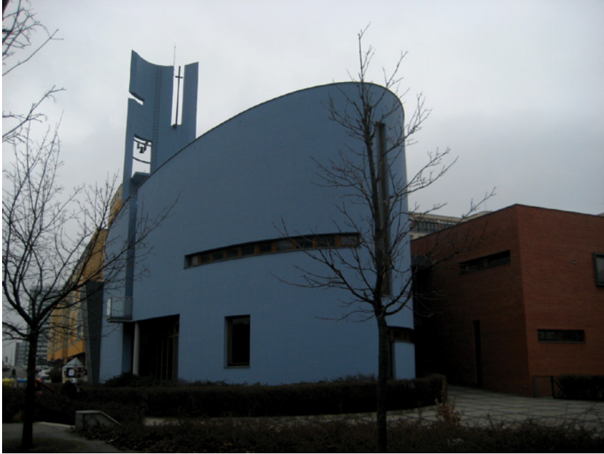
FIGURE 1.5 St Prokop, Prague-Nové Butovice, Czech Republic (Zdenek Jiran, Michal Kohout, 2001)
