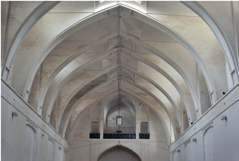
Fig. 12: Transverse vaulting in the west prayer hall added to the congregational mosque at Yazd, 765–77/1364–76. Author's photo.
