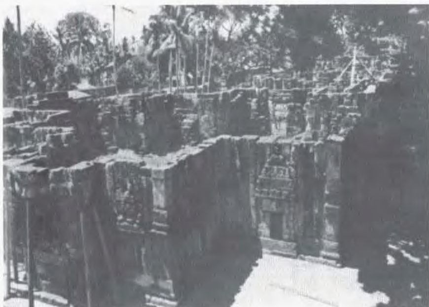
Photo 17. Mock-up or trial reconstruction of a horizontal section of the wall of the Śiva temple (OD 13297, reproduced from Djāwā 20 (1940))
