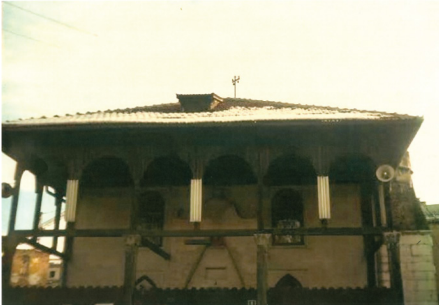
FIGURE 18 Magribija mosque. This photograph was taken before the start of the reconstruction work on the mosque, which has since been refurbished, and its old and rare wooden minaret, which was knocked down by a shell, has been replaced by a new stone one.
