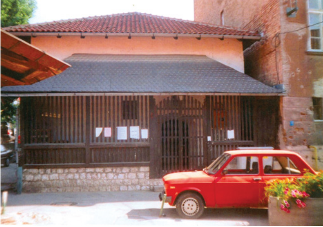
FIGURE 25 Sarajevo's Tabački Mesdžid (the tanners' mosque). Although refurbished and redecorated on many occasions since it was built in 1591, Sarajevo's Tabački Mesdžid is still very much the same today. It is situated in the back of Tabaci, the tanners' street, on the right bank of the river Miljacka (see Fig. 19). Just like the tanneries used to be separate from other crafts' quarters, partly because of their need to be located near water, but mainly because of the bad smell they produced, so did the tanners usually have to have a separate mosque for their own needs, as the odour of their clothes would offend other worshippers in an ordinary mosque.
