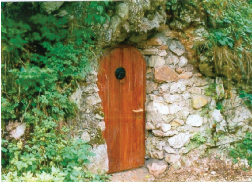
FIGURE 24 The door recently fitted to the dervish cave in Šehova Korija, as part of the project for its protection as a historical monument.
