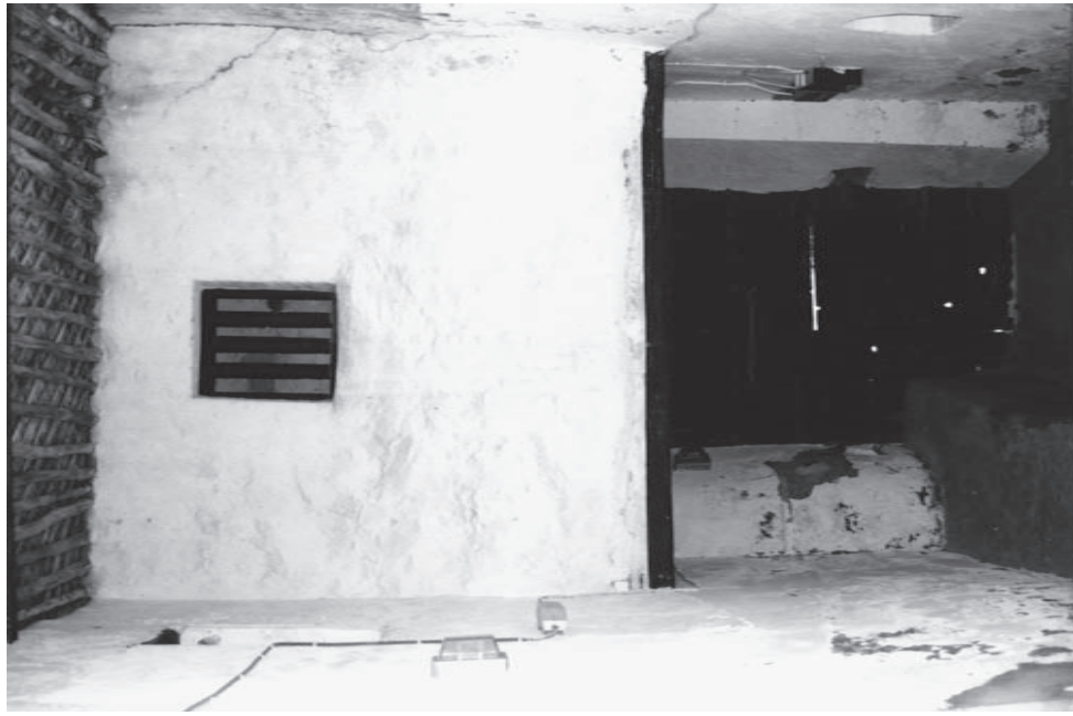
82. The same entrance from the inside.
