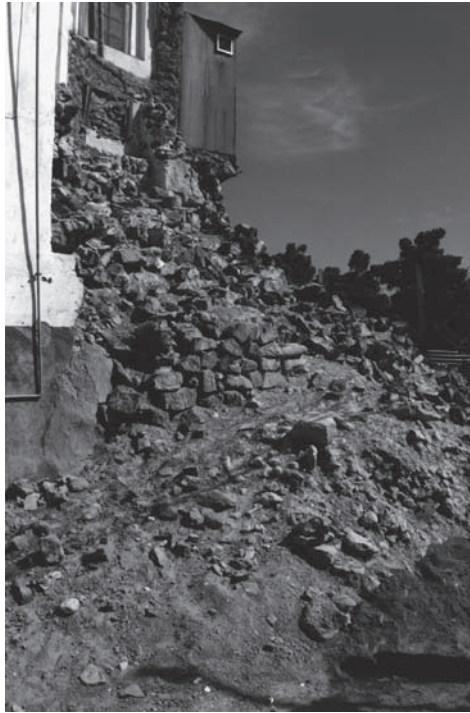
190. The tower on the southeast corner was reduced to rubble.
