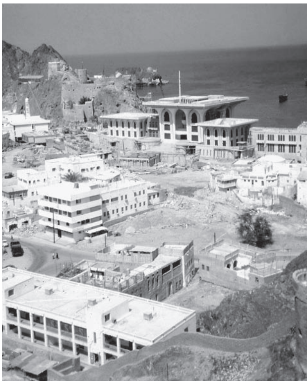
110. The new Qasr al-'Alam palace under construction in 1975.
