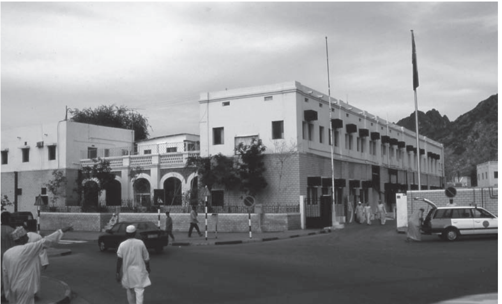
181. Al-Rahmah Hospital in 1996, shortly before its demolition.
