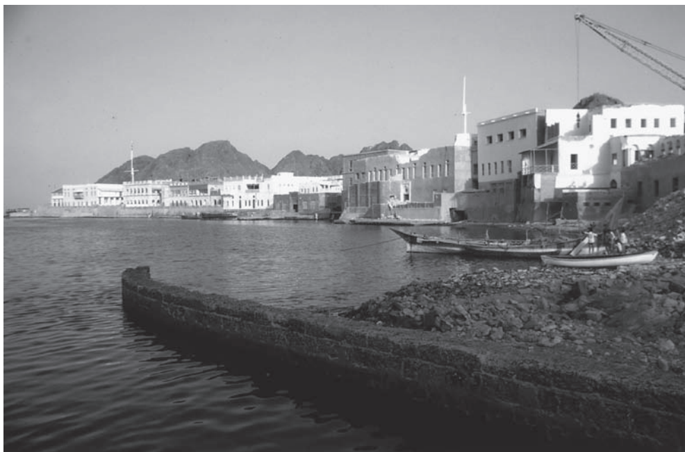
109. The early stages of the demolition of Bayt al-'Alam in 1971.
