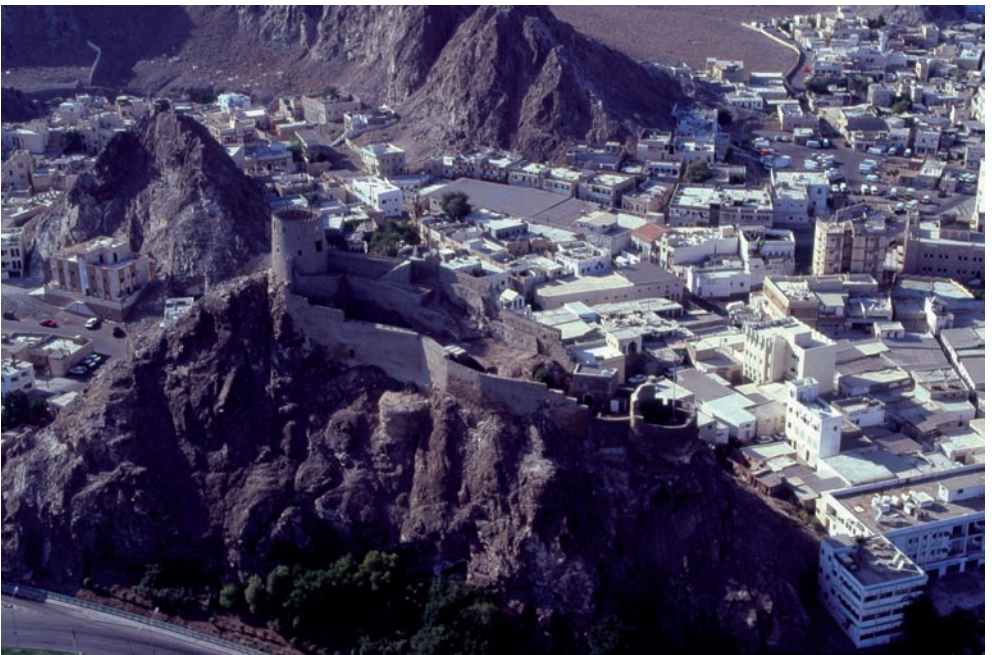
44. Matrah fort in 1998. This view shows the narrow space between the curtain walls and the two watchtowers at either end that formed the original fortifications on the site.
