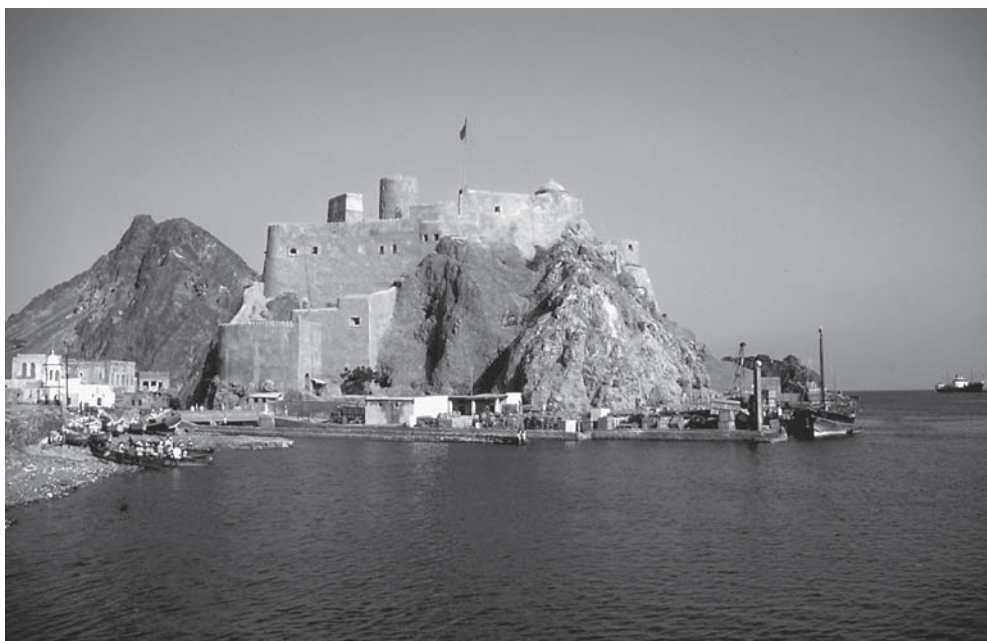
78. The fort in 1970, with the busy Khawr Jetty, constructed in the mid-20th century, beneath it.
