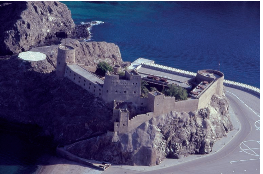
19. An aerial view of Fort al-Jalali, illustrating the narrowness of the gun deck and the staircase to the original entrance.
