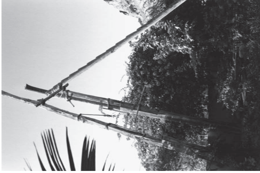
144. The wooden superstructure or turkbah of a zajirah well, still standing in 1995.
