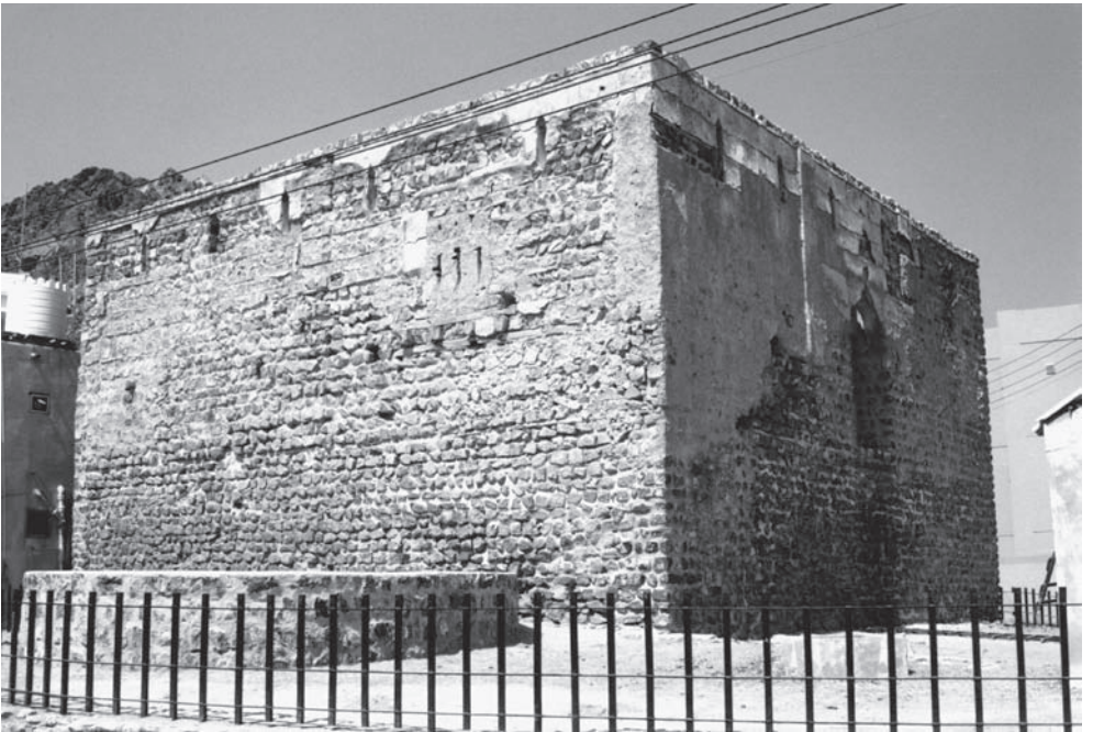
94. The fort from another angle with the disused well in the foreground.
