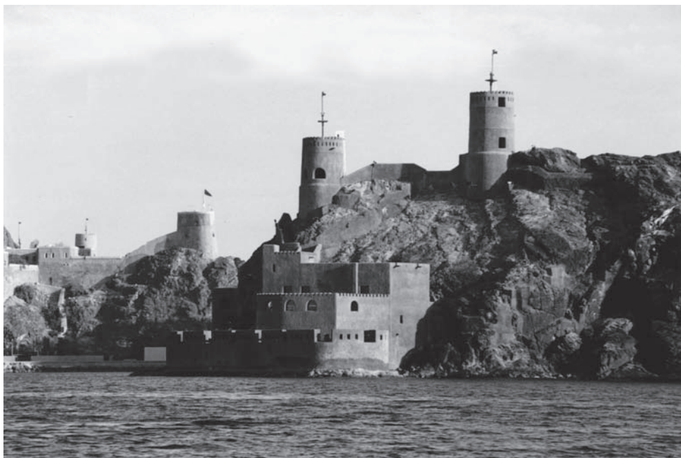
90. A 1996 view of the defenses from outside the harbor entrance.
