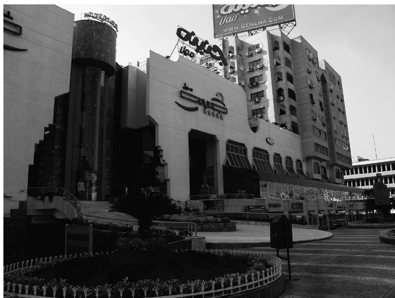
Fig. 86. Gencina Façade, January 2006.
