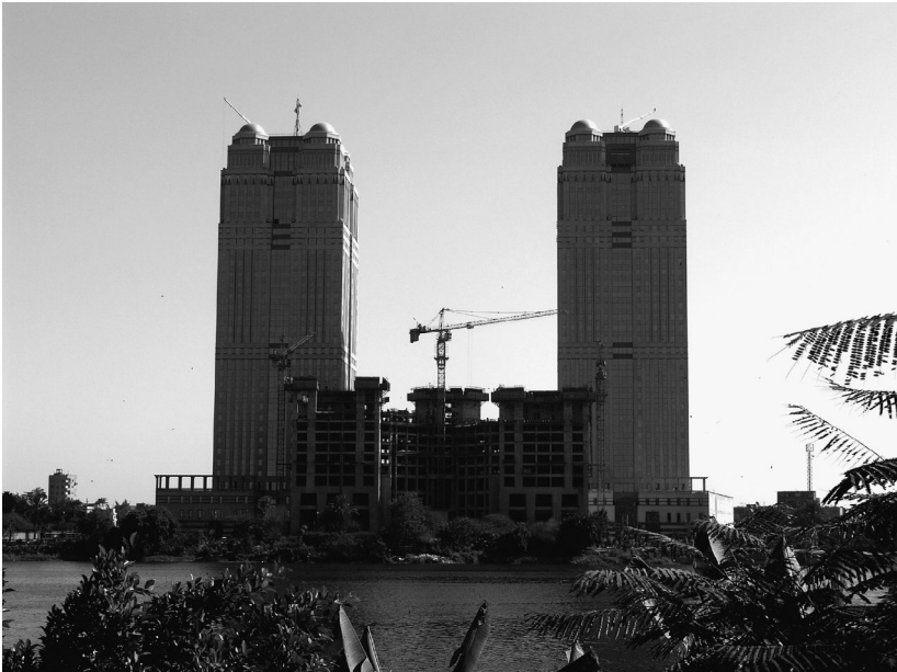
Fig. 10. Nile Towers, Bulaq, view from Zamalek.
