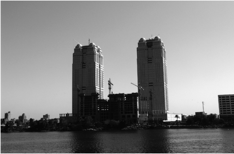
Fig. 4. Nile Towers, Bulaq, view from Zamalek.
