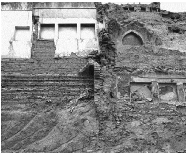
Fig. 10. Site excavated for new construction south of Masjid-i Malik; medieval collapsed arch at bottom, centre.
