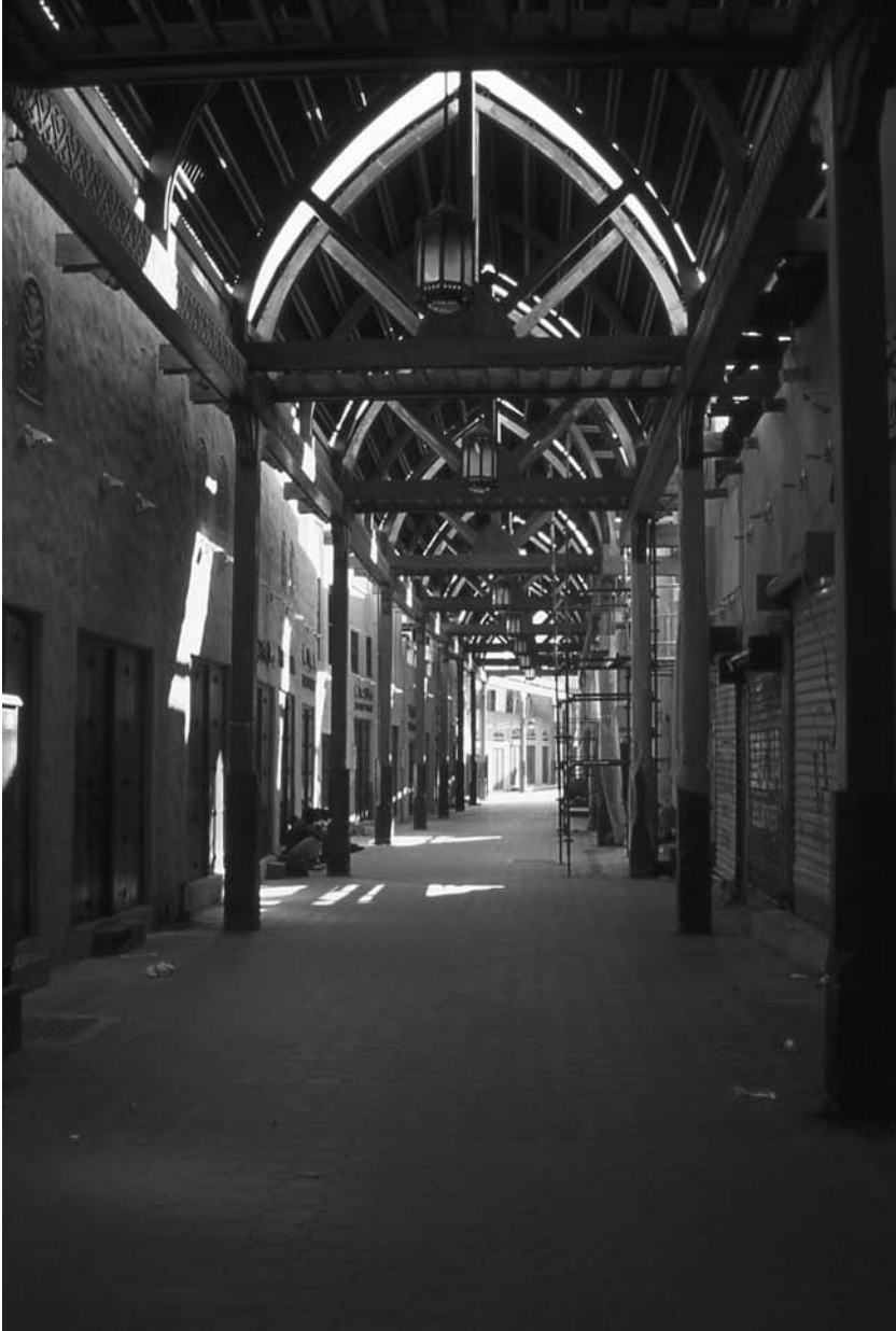
Fig. 3. Grand Souq with wooden roof structure.
