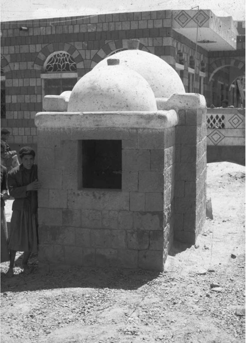
Fig. 18. A street corner cistern.
