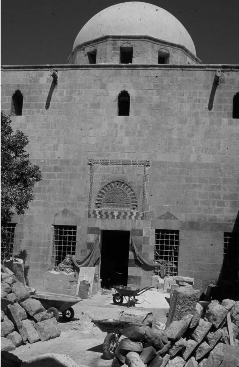
Fig. 9. Front qa'a of the Maktabi house (sixteenth century), during restoration.
