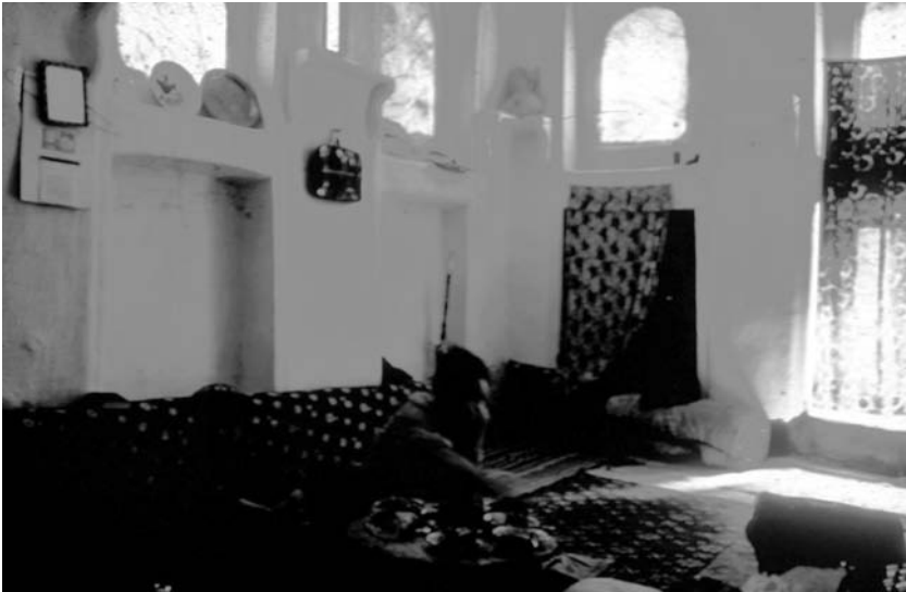
Fig. 14. A typical room with gypsum in the upper windows.
