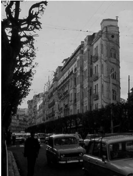
Fig. 3. The stair used as a corner solution in rue Michelet today Didouche Mourad.
