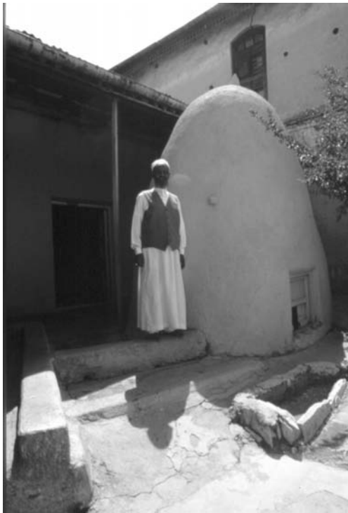
Fig. 2. A courtyard house.
