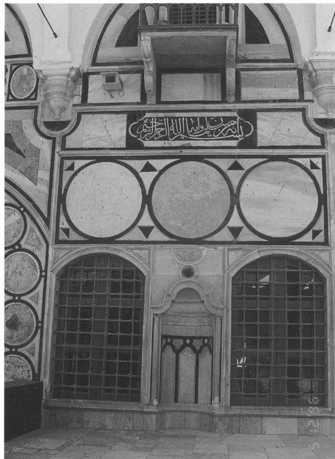
Fig. P2 Jazzar Mosque. North wall right of main gate
